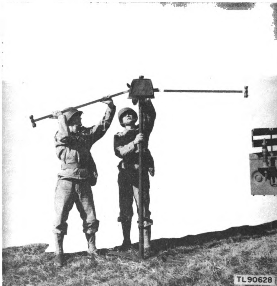
Figure 25. Placing crossarms in mast.
