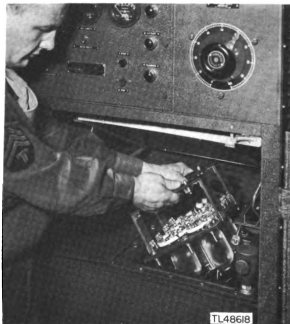
Figure 4-8. Removing keyer tubes.
