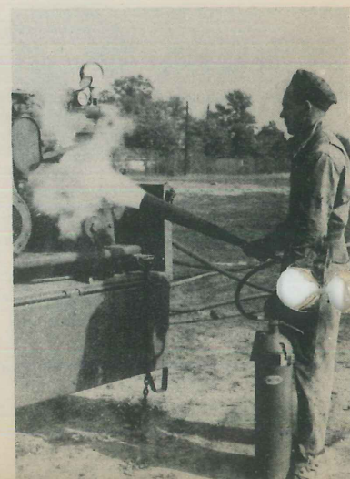
Picture at right shows use of carbon dioxide extinguisher on a gasoline engine. Note that this vapor is aimed above the engine. View below shows carbon tetrachloride extinguisher which is operated by turning handle and then pumping fluid at base of flame. This type has no trigger and no compressed air chamber.
