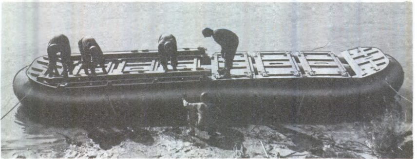
Step 5. Female sections of saddle beams in position
