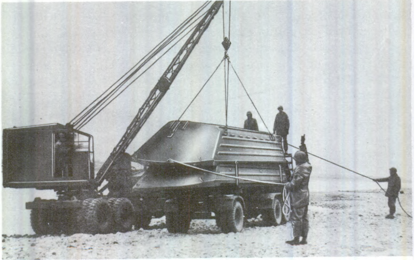
Step 1. Crane attached to half-ponton
