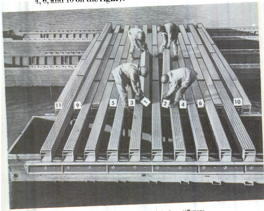
Step 13. Laying balk across interior stiffeners
