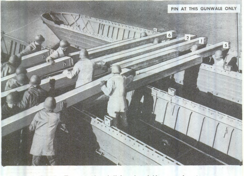
Step 2. Four near-shore balk have been laid on second ponton
