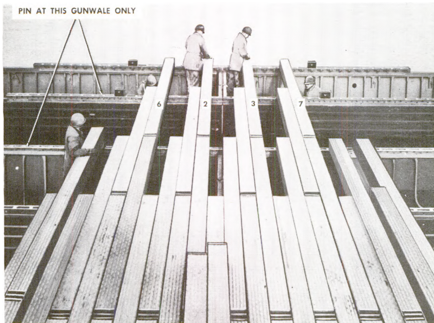
Step 4. Adding balk to new ponton
