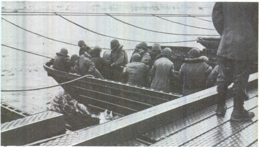
② New ponton in approximate final position Figure 97. Replacement of damaged ponton.
