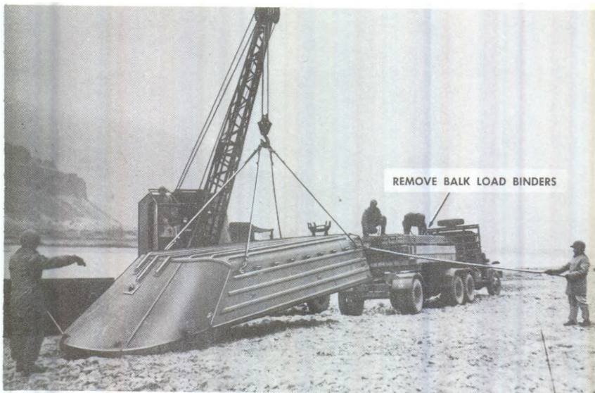
Step 3. Unloading second half-ponton
