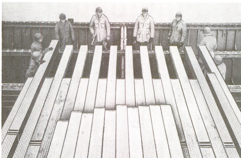
Step 2. Ponton alongside bridge
