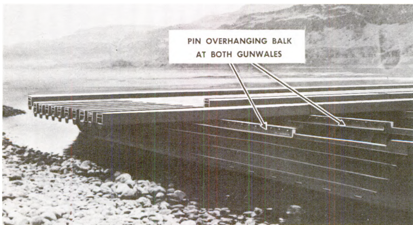
Step 2. Eleven near-shore balk in place and pinned
