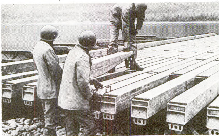
Step 5. Placing tapered balk
