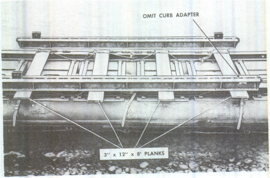
Step 7. Temporary supporting float completed
