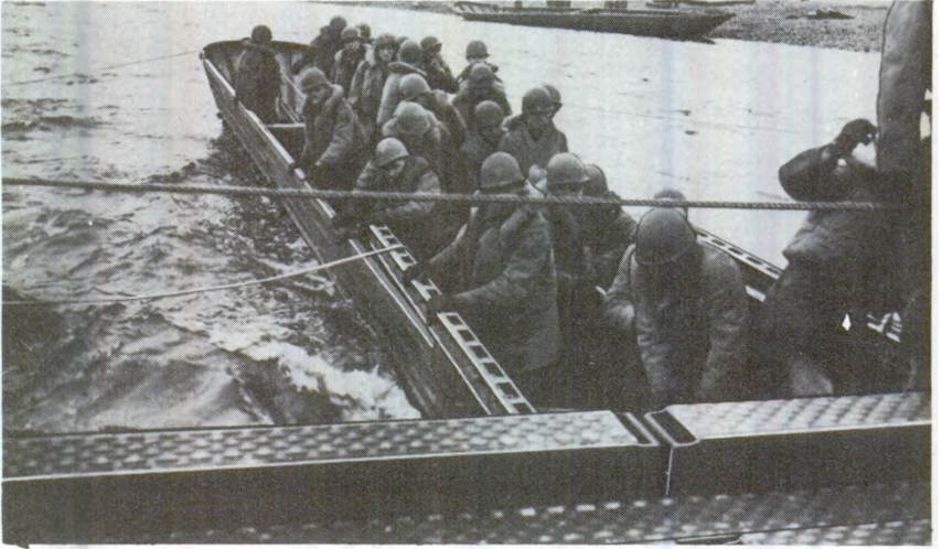
① New ponton being pulled under removable gunwale from downstream side
