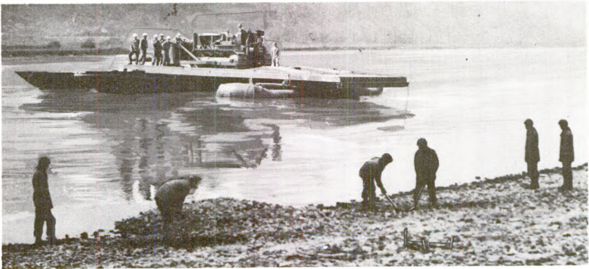
Step 3. Preparing temporary landing stage
