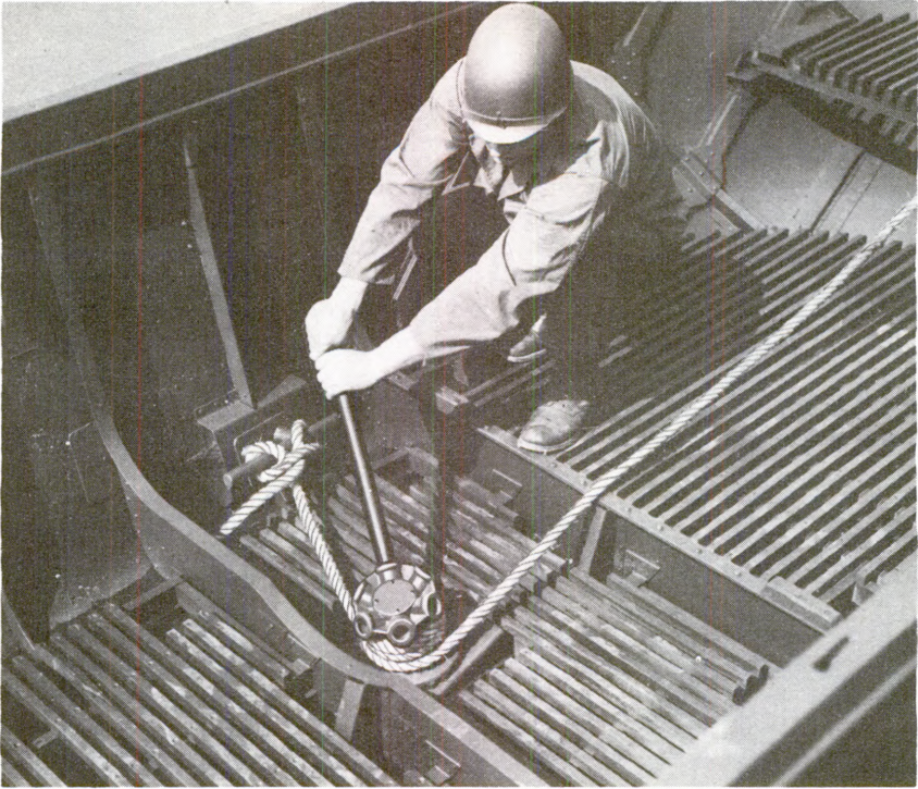
Step 6. Alining ponton by adjusting bridle line
