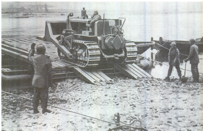
Step 4. Unloading bulldozer from moored end section
