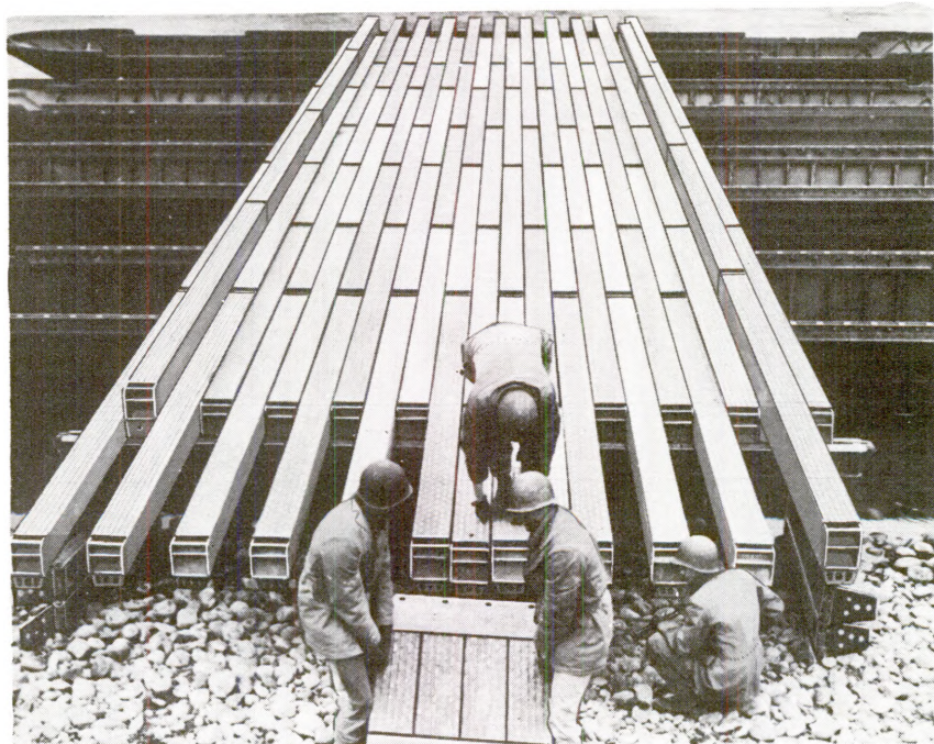
Step 6. Placing ramp
