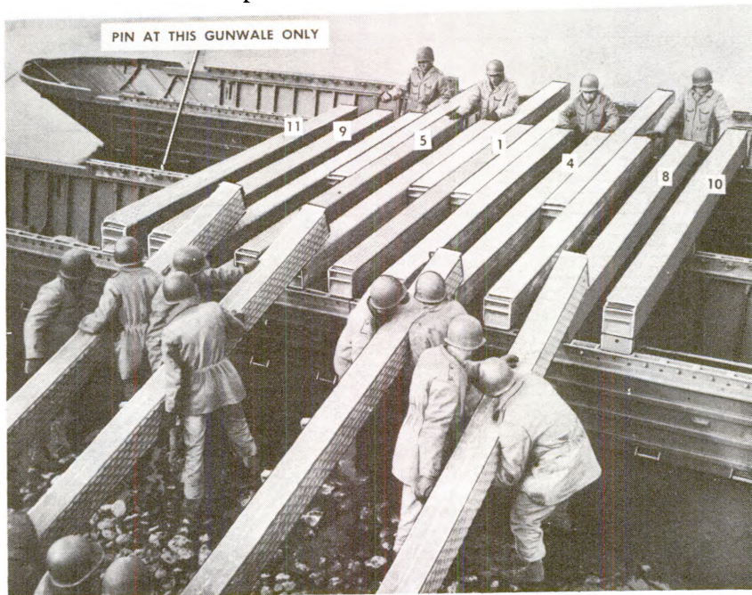
Step 3. Laying remainder of far-shore balk on first ponton
