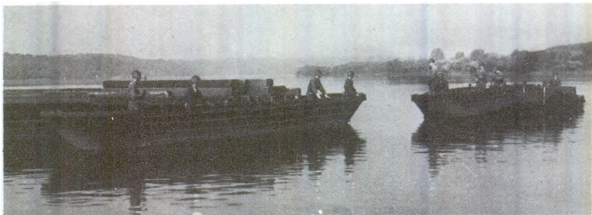
Step 1. Ponton being moved into position
