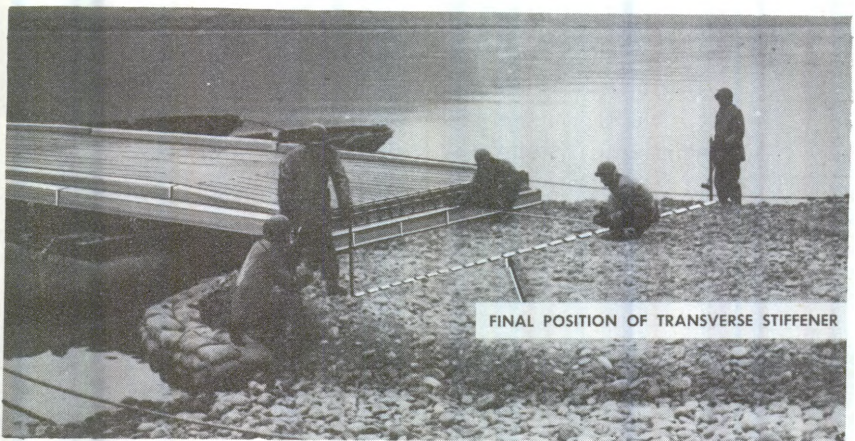
Step 2. Establishing final position of transverse stiffener
