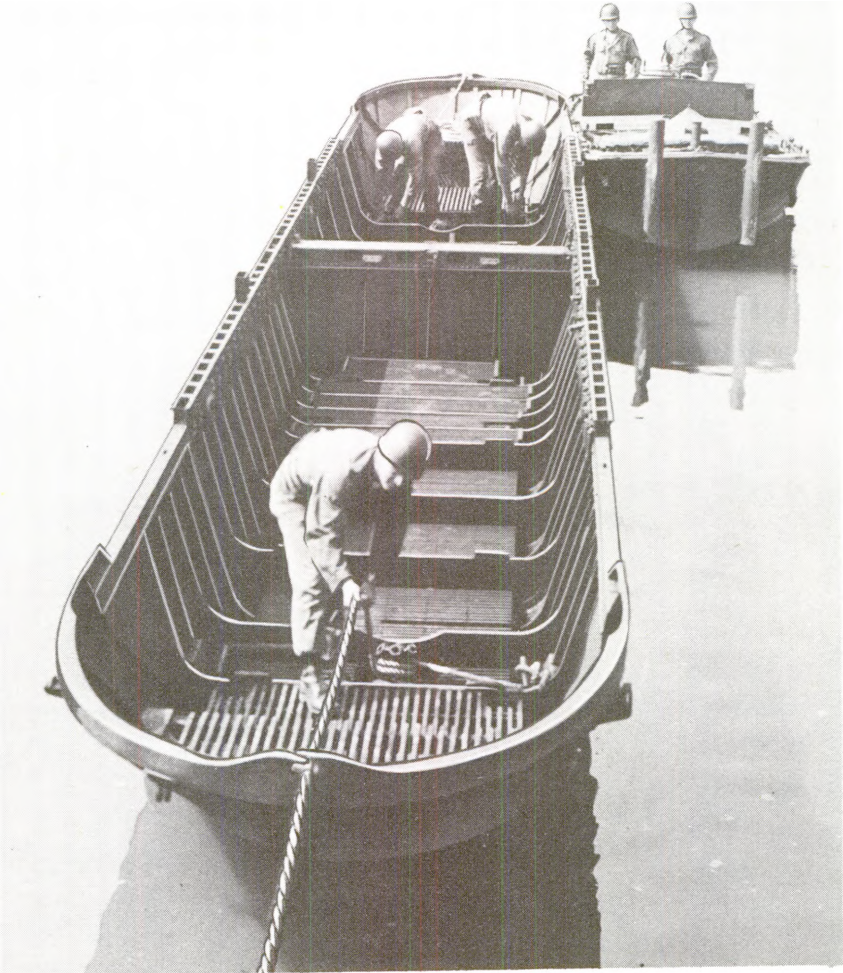
Step 6. Bridge erection boat moored to downstream half-ponton
