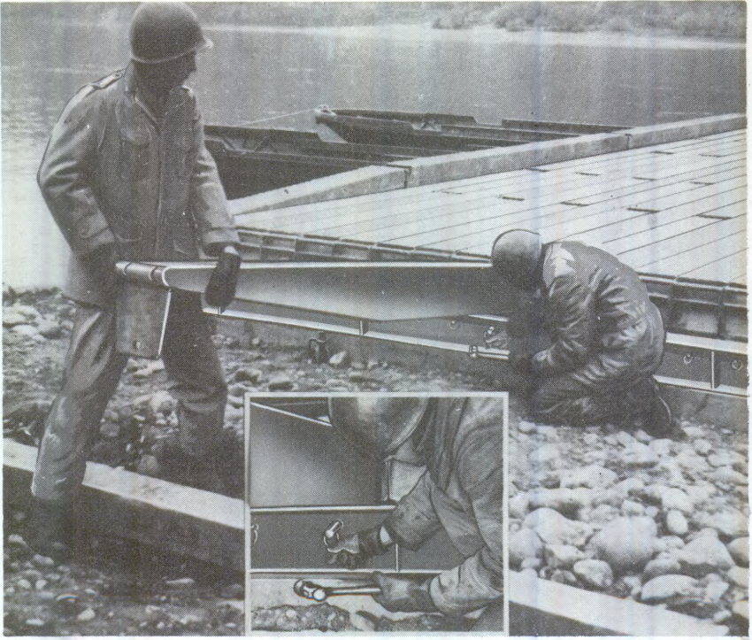
Step 5. Pinning tapered balk to transverse stiffener
