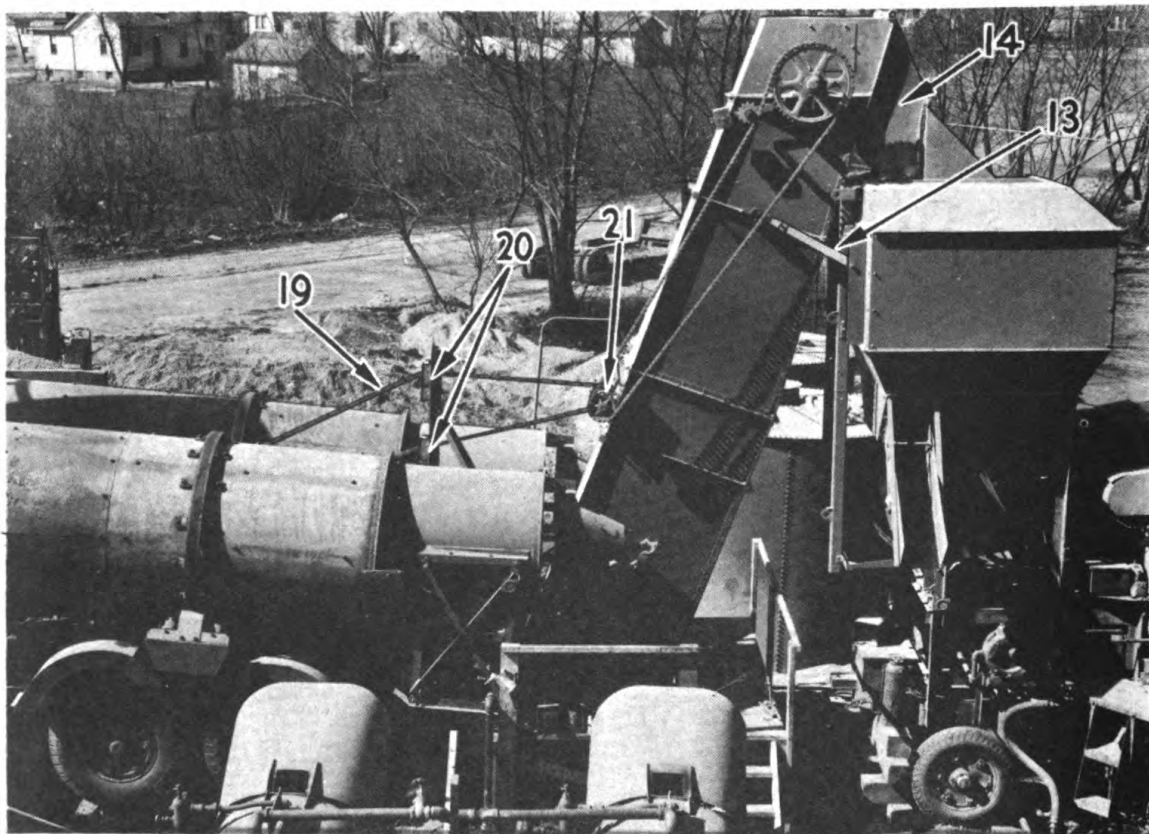
FIG. 58 - "HOT ELEVATOR IN OPERATING POSITION WITH PUSH ARMS AND DRIVE CHAINS INSTALLED.
