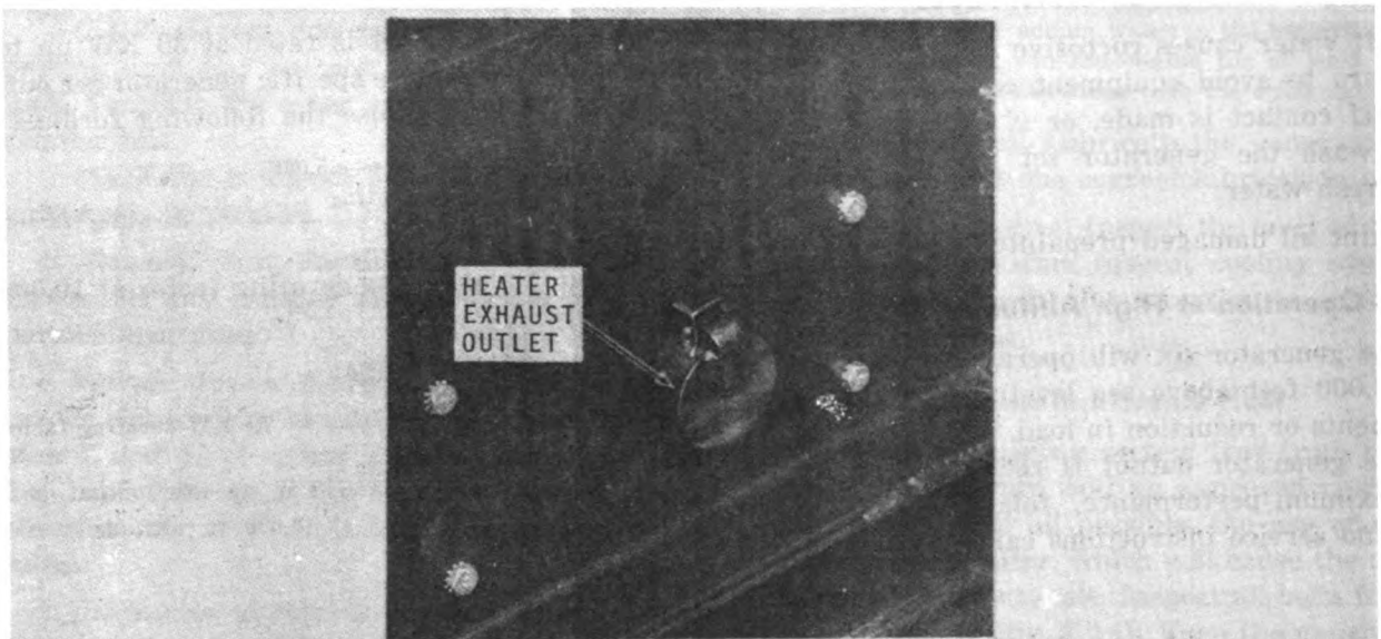
A. HEATER EXHAUST OUTLET
