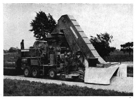
Figure 2. Barber-Greene Paving Loader and Heavy Duty Mixer in Travel Plant Operation.
