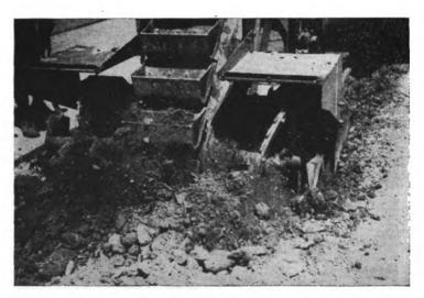
Figure 29. Preparing the sub-base between two existing concrete strips. The scarified dirt and stones were loaded continuously into trucks without halting traffic.
