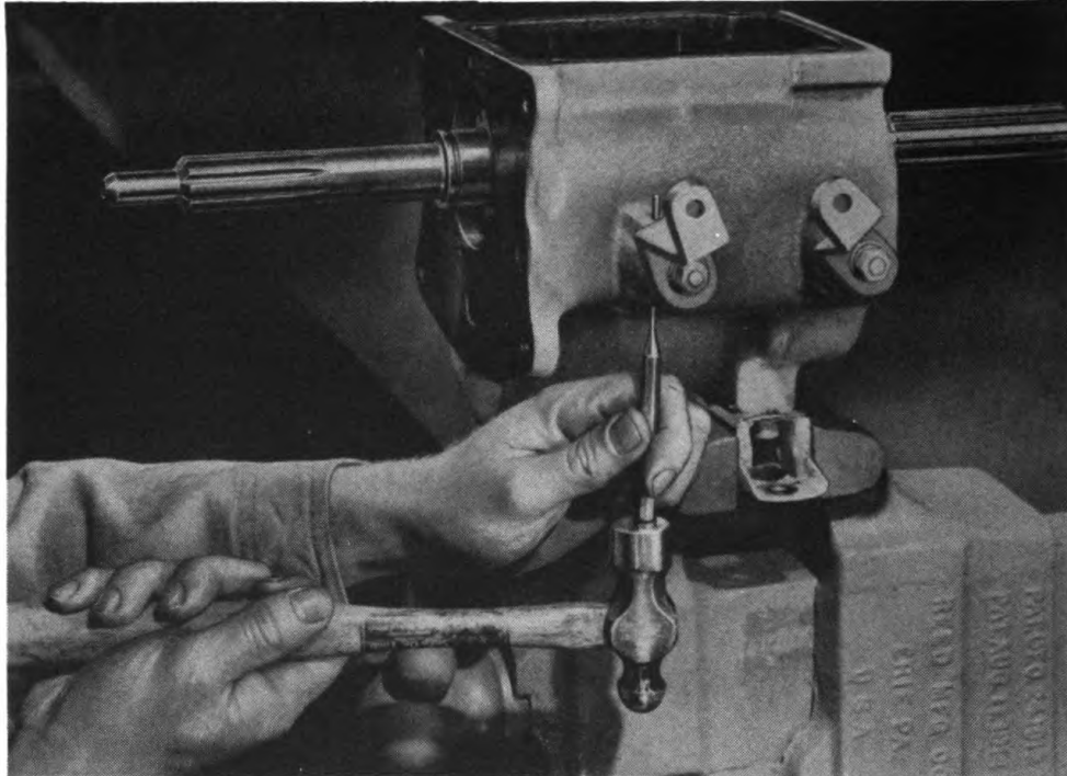
Figure 11—Shift Lever Shaft Pins Removal
