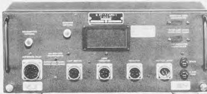
Transmitter Receiver RT-7/APN-1 On Mounting Base MT-14/ARN-1
