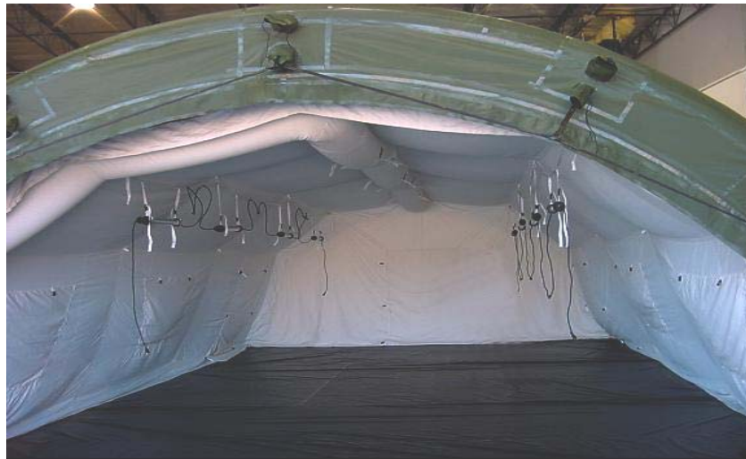
Figure 22. Lighting Kit Installed.
