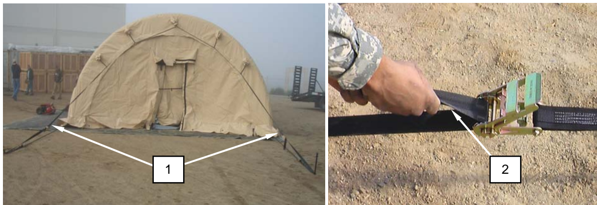
Figure 10. Removing Slack from Upper Ratchet External Bracing Straps.
