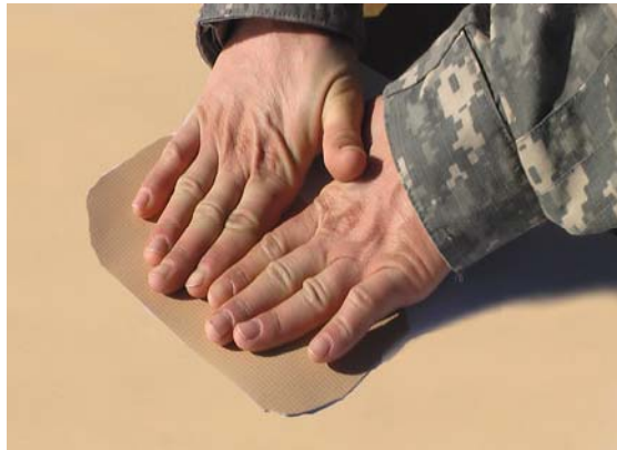
Figure 14. Remove Air Pockets from Patch.
