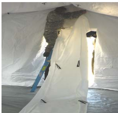
Figure 1. Lay Out Plenum for Patch Repair.
