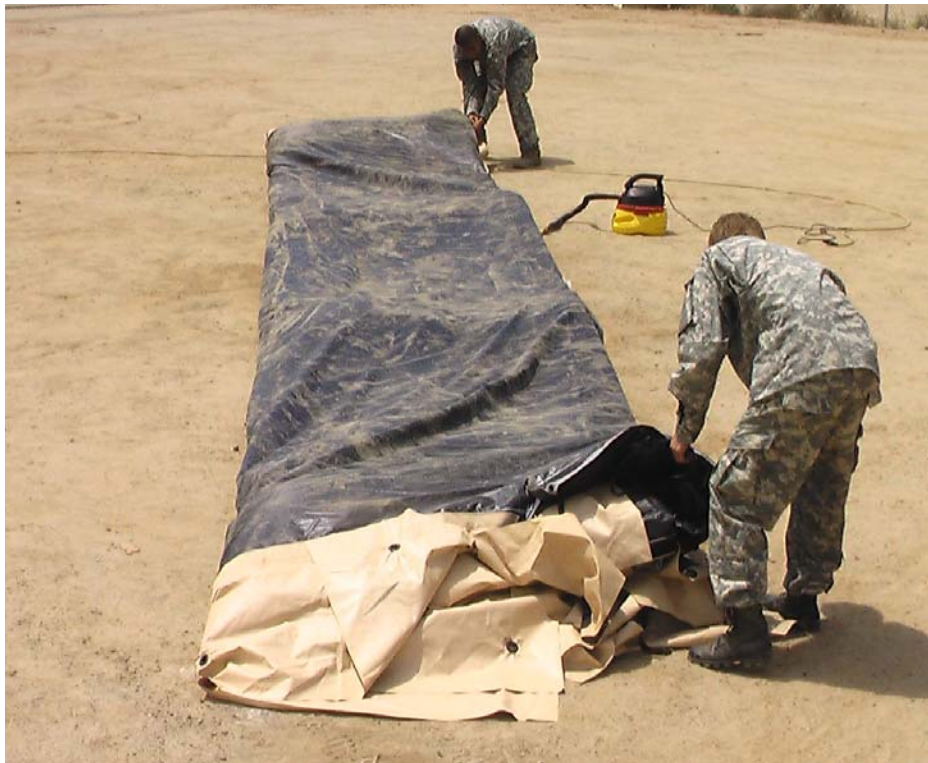
Figure 37. Second Fold of TEMPER, Air-Supported Shelter.
