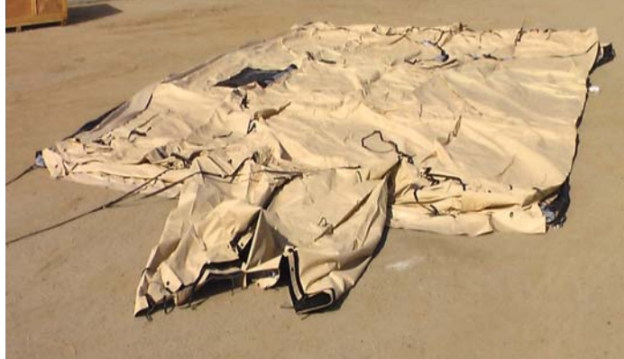
Figure 7. Unfold TEMPER, Air-Supported.
