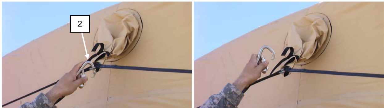
Figure 3. Releasing the Carabineers from the External Tensioning Snout Securing Loop.
