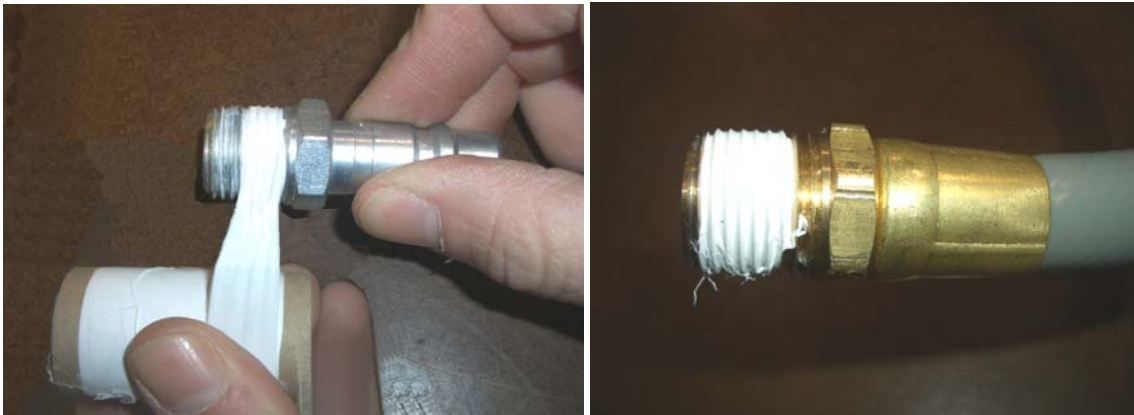
Figure 6. Wrap Threads with Sealant Tape.
