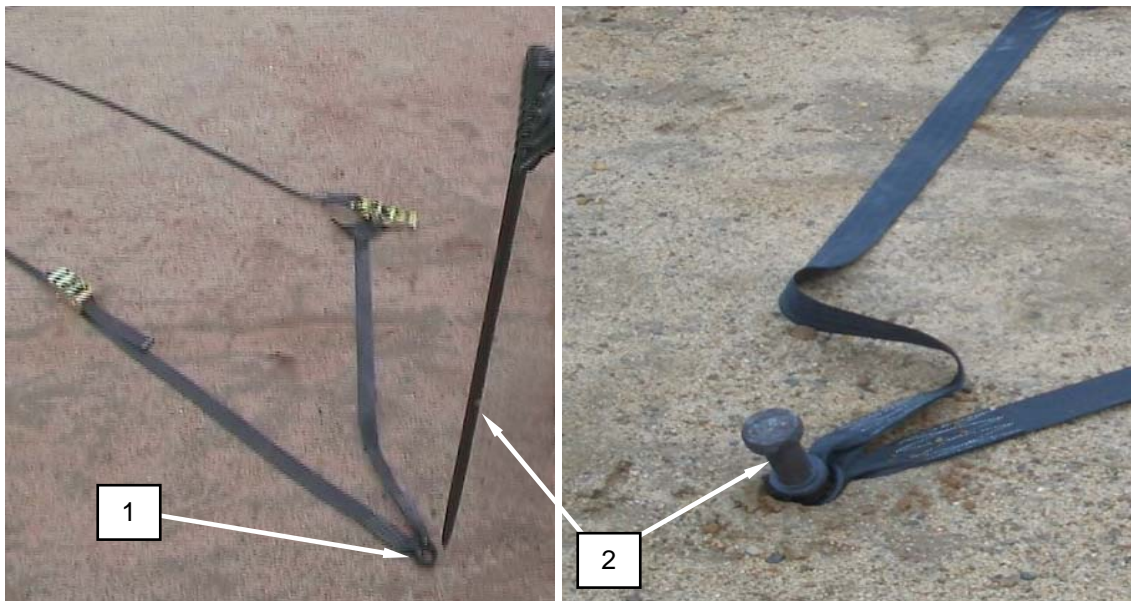
Figure 8. Position Bracing Strap End Rings.
