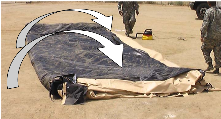
Figure 36. First Fold of TEMPER, Air-Supported Shelter.
