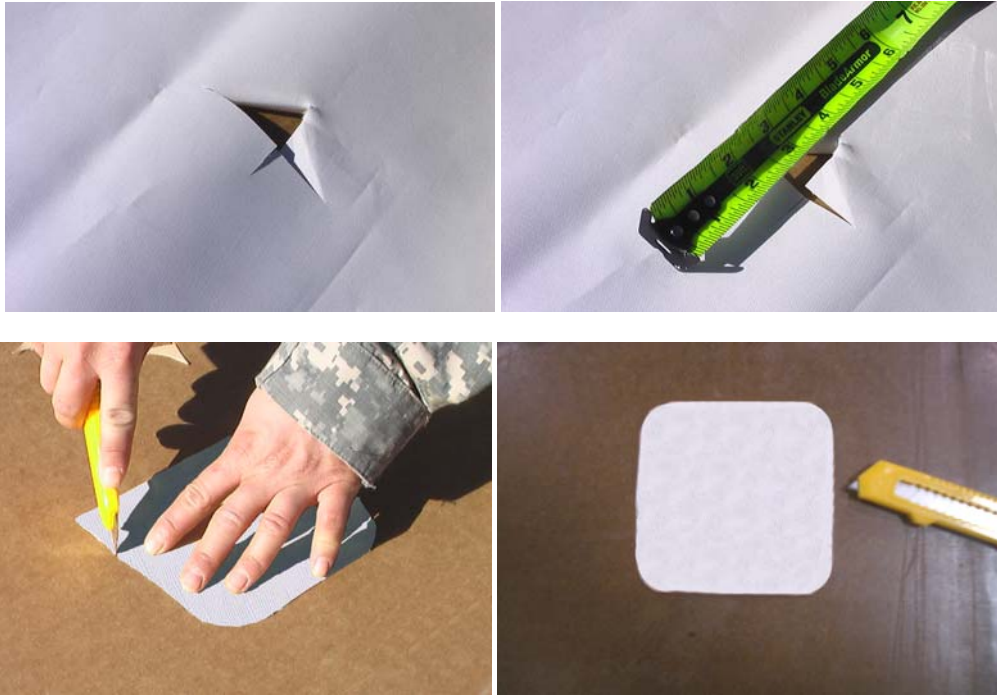
Figure 7. Measure and Cut Patch Material.
