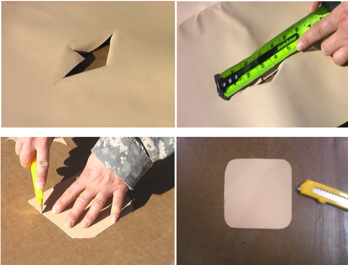
Figure 3. Measure and Cut Temporary Patch.
