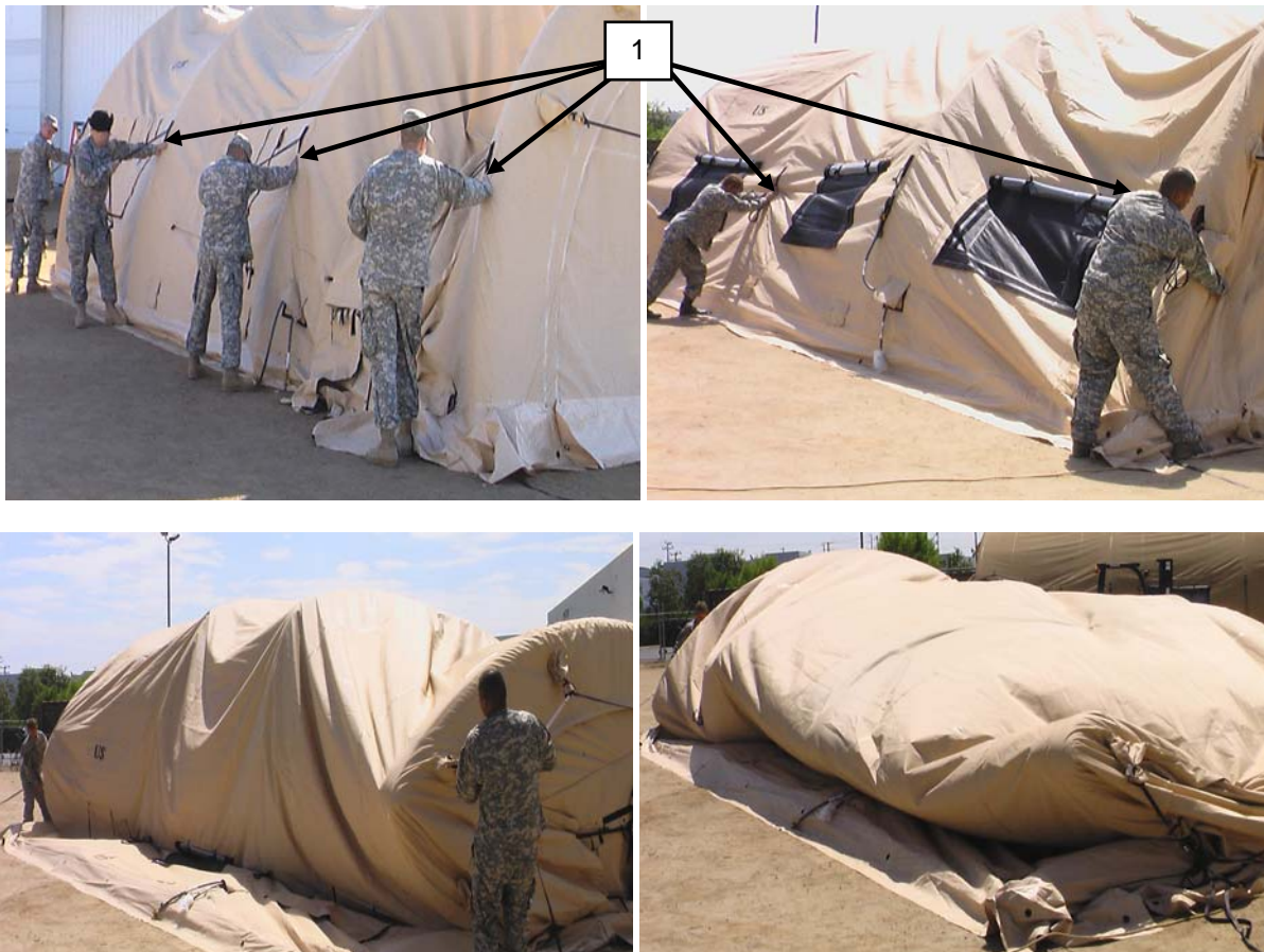
Figure 31. Knuckle Over the TEMPER, Air-Supported Shelter.
