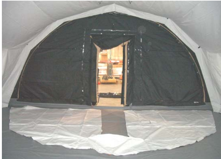
Figure 18. Lay Out Liner End Section.
