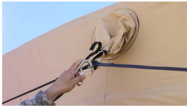
Figure 5. Securing the Ratchet Snow Strap Carabineer.
