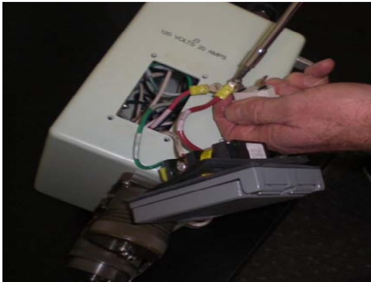
Figure 16. Connecting Circuit Breaker Wiring.
