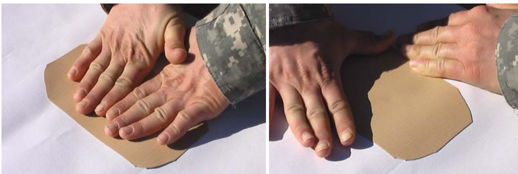
Figure 5. Main Liner Patch Repair.
