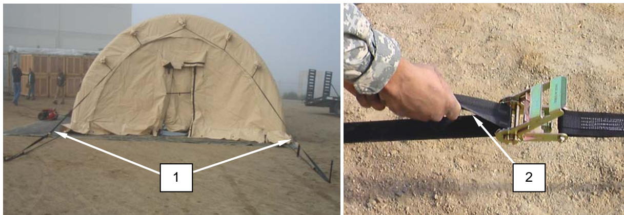
Figure 12. Removing Slack from Upper Ratchet External Bracing Straps.
