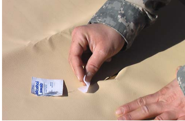
Figure 8. Preparing Damaged Area with Alcohol Prep Pad.
