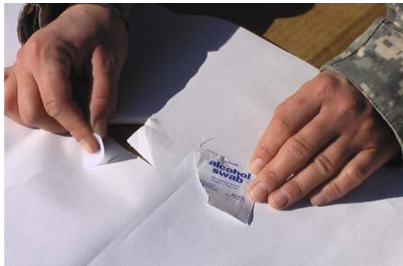
Figure 9. Prepare Adhesive Patch Area.
