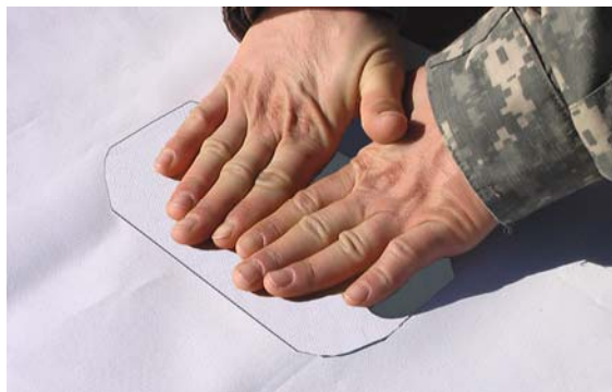
Figure 14. Remove Air Pockets from Patch.
