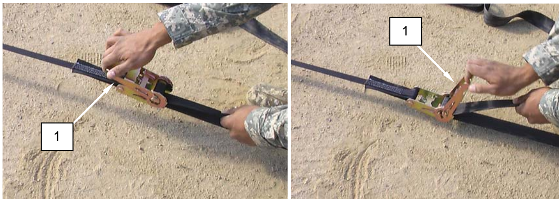
Figure 12. Tighten Upper Ratchet External Bracing Strap with Tensioning Ratchet.
