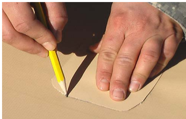
Figure 10. Trace Patch Perimeter with Pencil.
