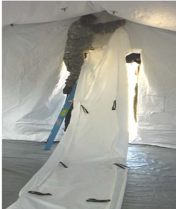
Figure 18. Prepare Plenum for Installation.
