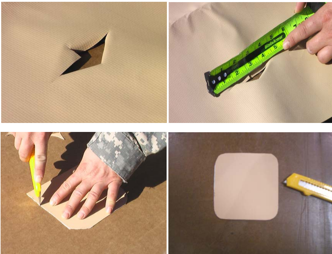
Figure 7. Measure and Cut Patch Material.
