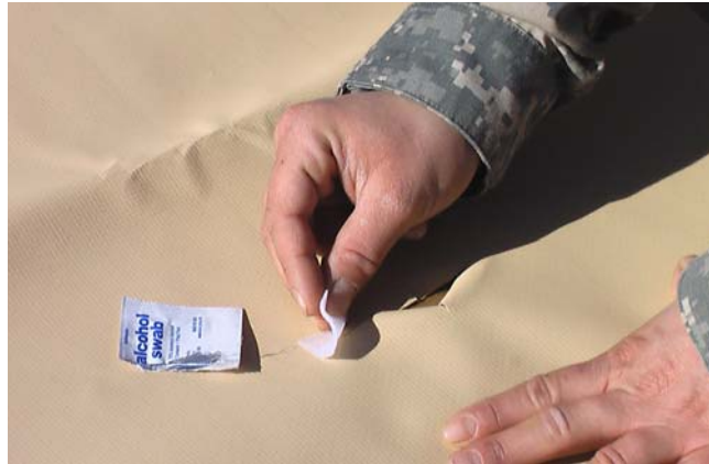
Figure 8. Preparing Damaged Area with Alcohol Prep Pad.
