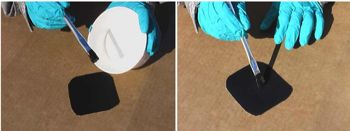
Figure 12. Apply Adhesive to Patch.
