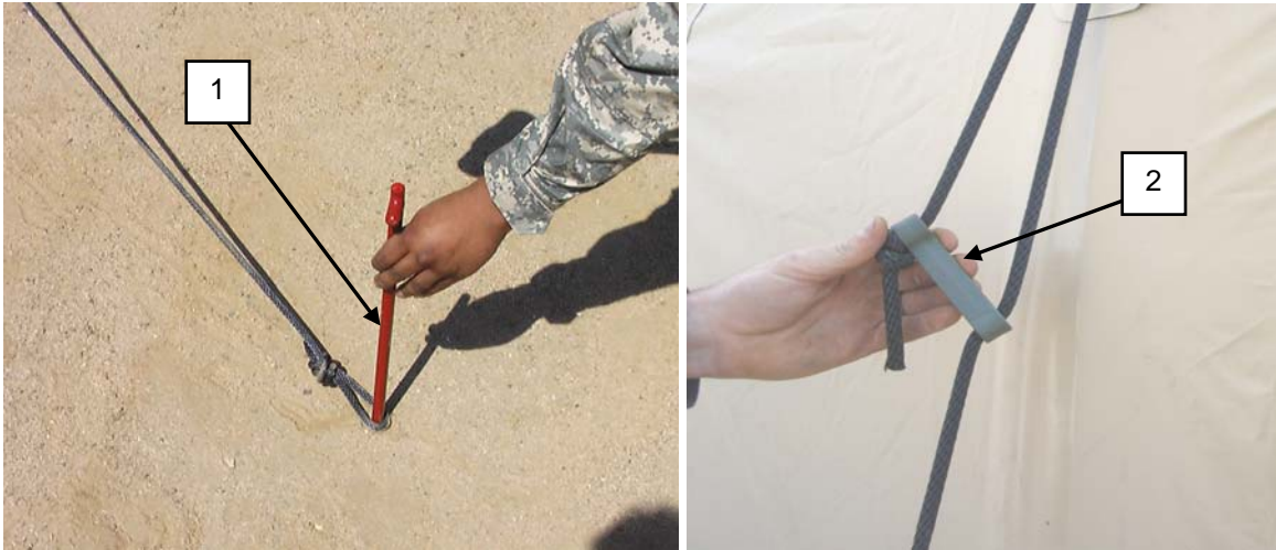
Figure 71. Staking Vestibule Guy Lines.
