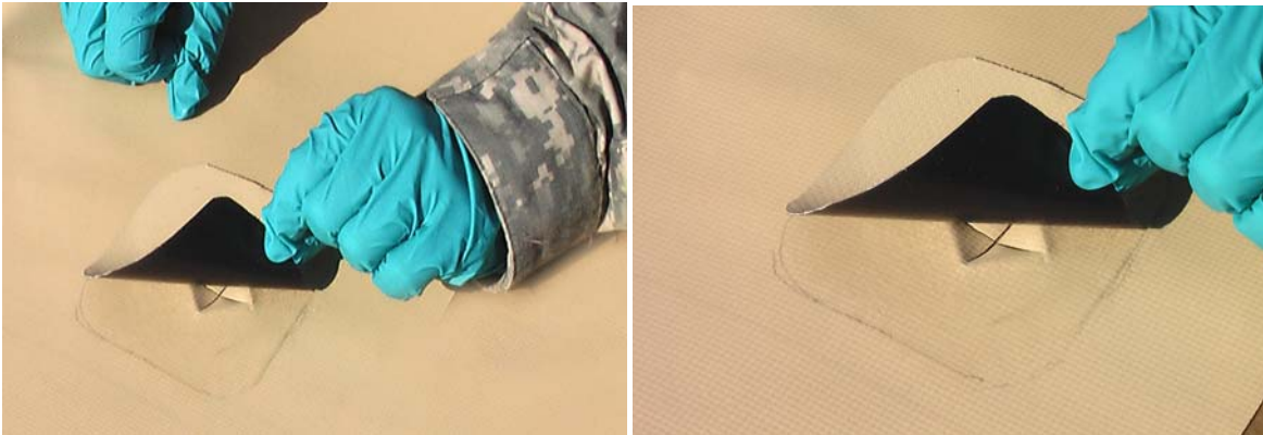
Figure 13. Apply Patch to Damaged Area.
