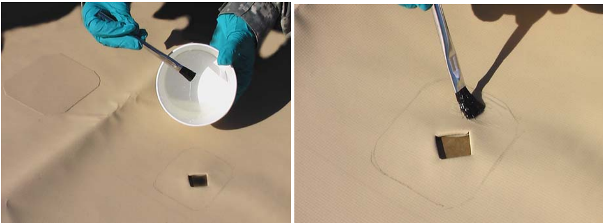
Figure 11. Apply Adhesive to Damaged Area.
