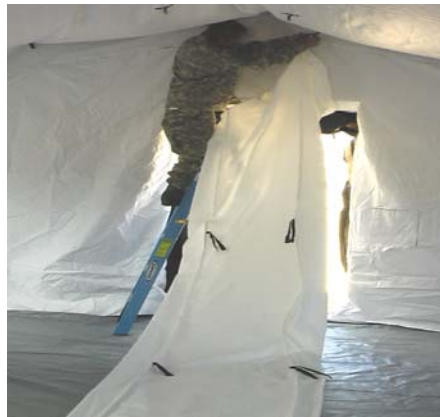
Figure 6. Lay Out Plenum for Patch Repair.
