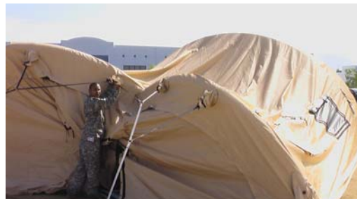
Figure 4. Airbeams Lifted Into Position.
