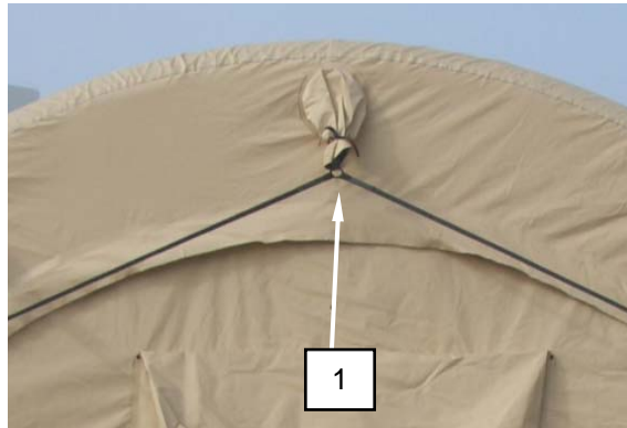
Figure 8. External Bracing Tensioned.
