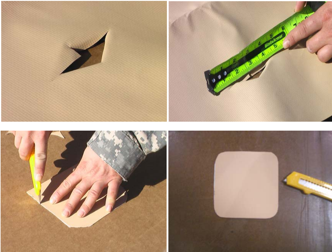
Figure 5. Measure and Cut Patch Material.
