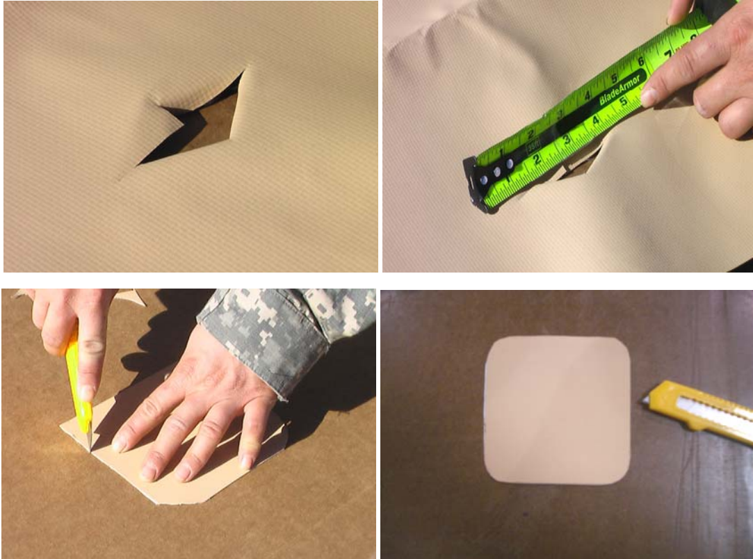
Figure 1. Measure and Cut Temporary Patch.
