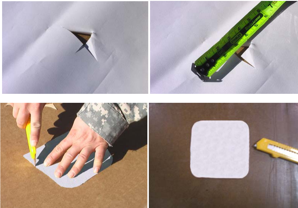
Figure 2. Measure and Cut Patch.
