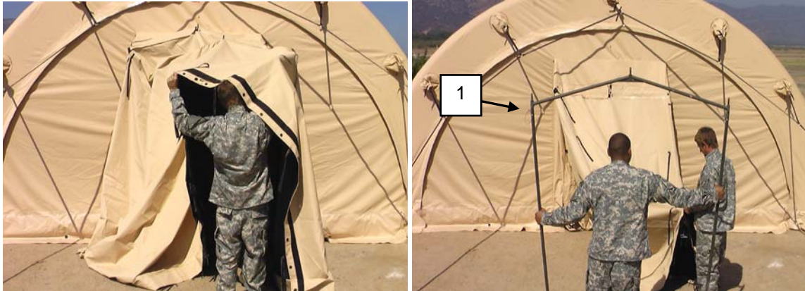
Figure 26. Remove Vestibule Frame Sections.
