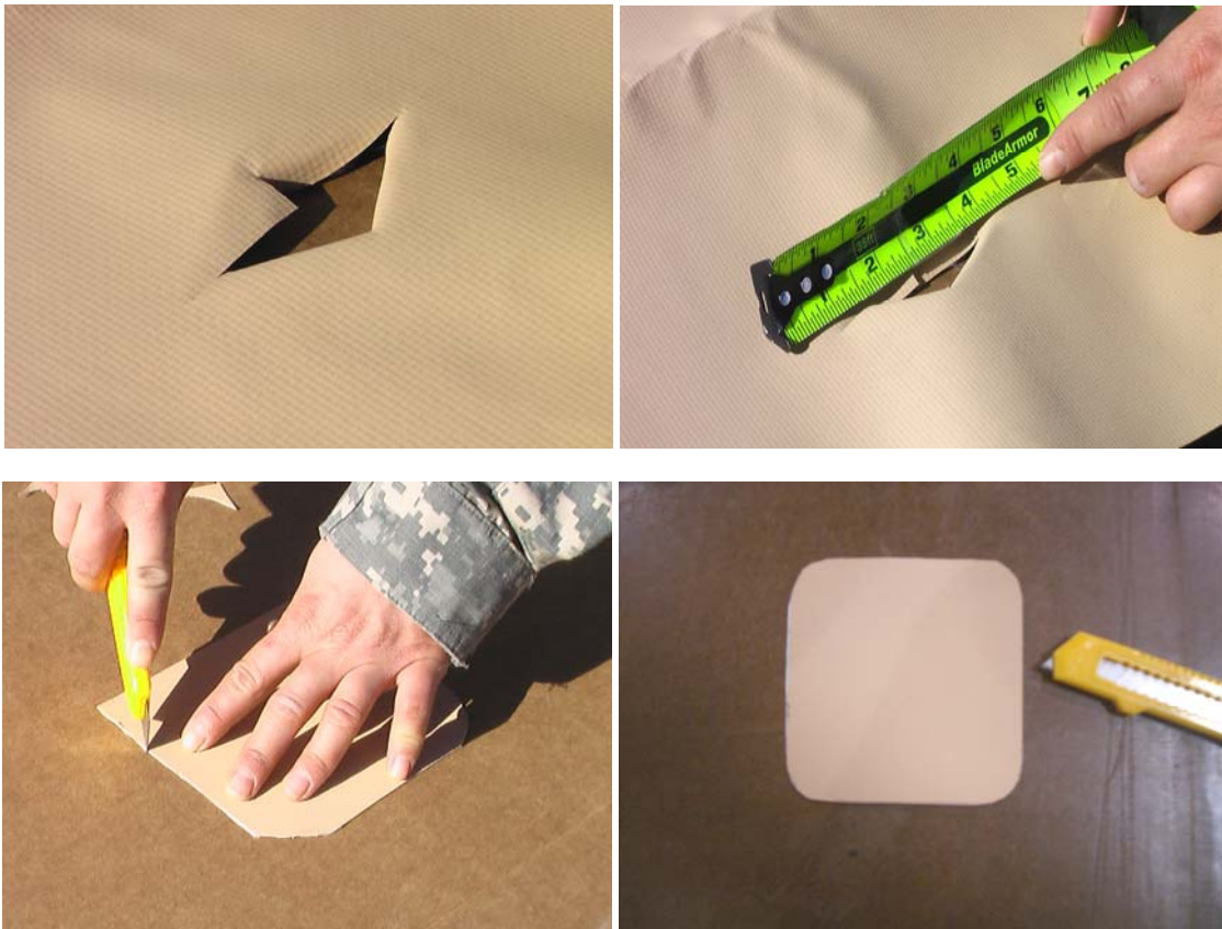
Figure 7. Measure and Cut Patch Material.
