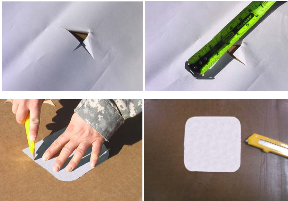
Figure 2. Measure and Cut Patch.
