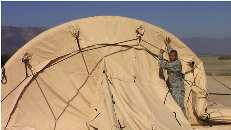
Figure 45. Assisting the End Air Beams into Position.
