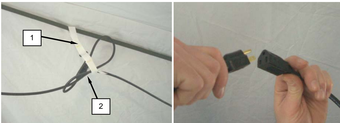
Figure 25. Disconnect Light Fixture Power Cords.
