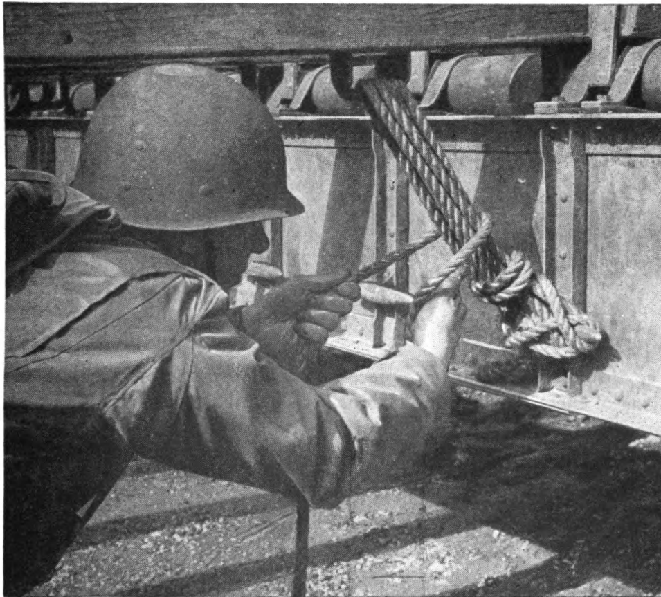
Figure 36. Lashing outside balk to transom
