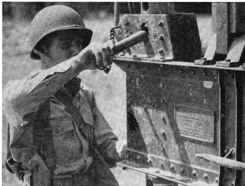
Figure 3. Pin being inserted in transom and column
