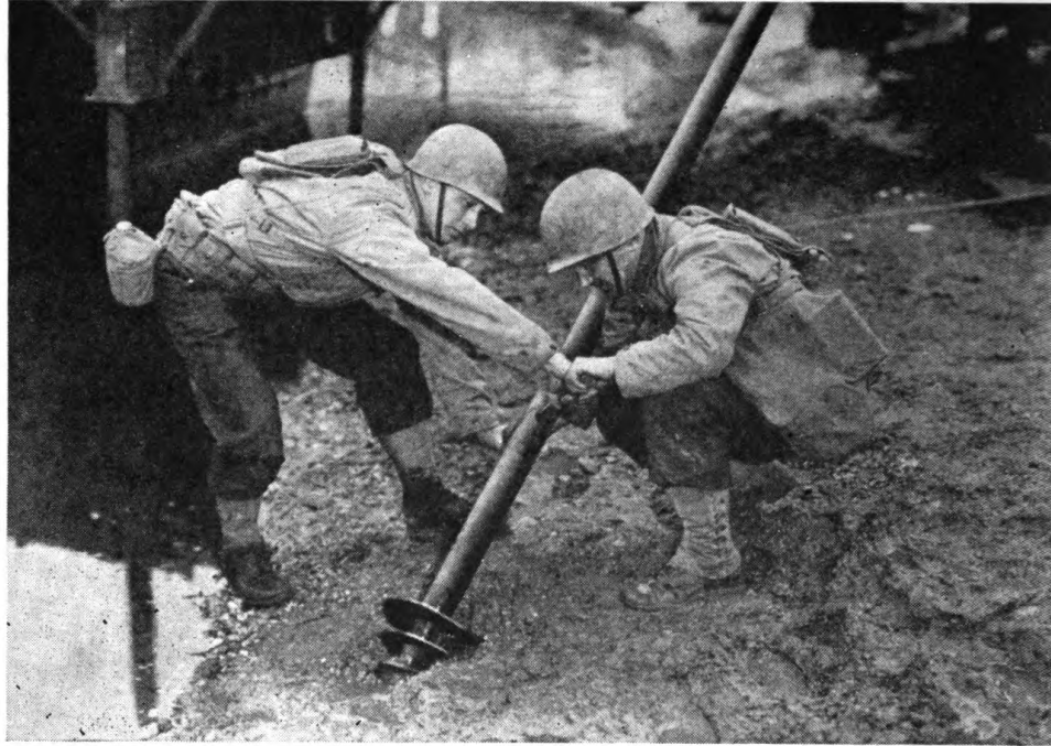
Figure 34. Screwing bracing strut shoe into ground
