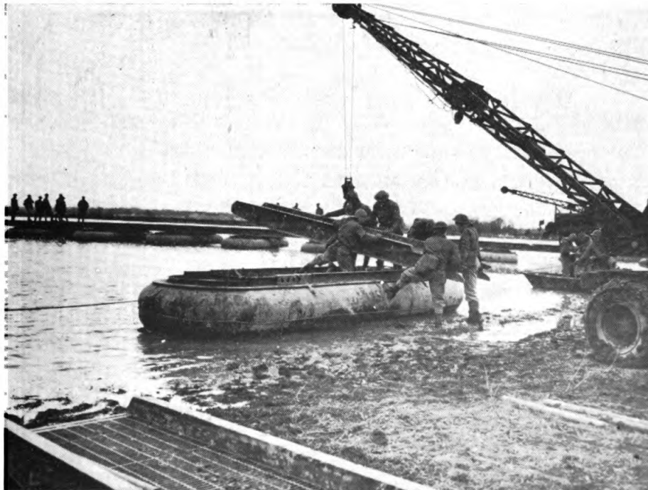
Figure 22. Placing treadways in assembling a ponton section.
