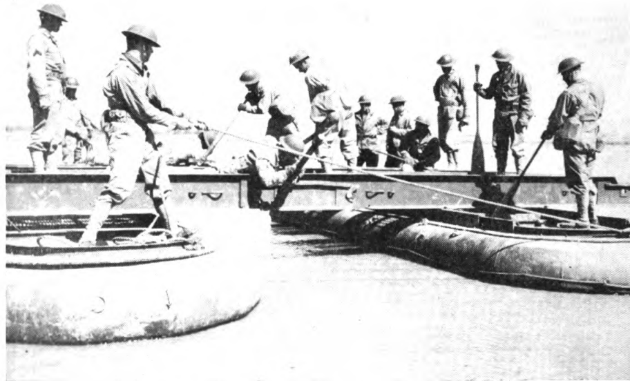
Figure 25. Installing connecting pins.
