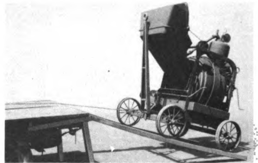
LOADING WITH RAMP & WINCH
