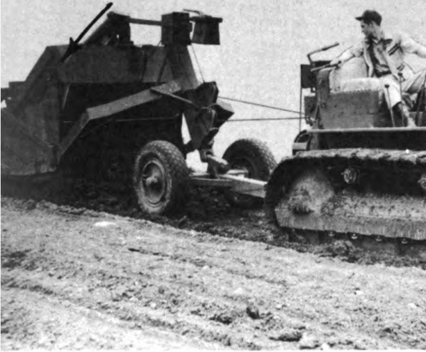
APRON RAISED TO FULL HEIGHT TO PERMIT DIRT TO FALL OUT
