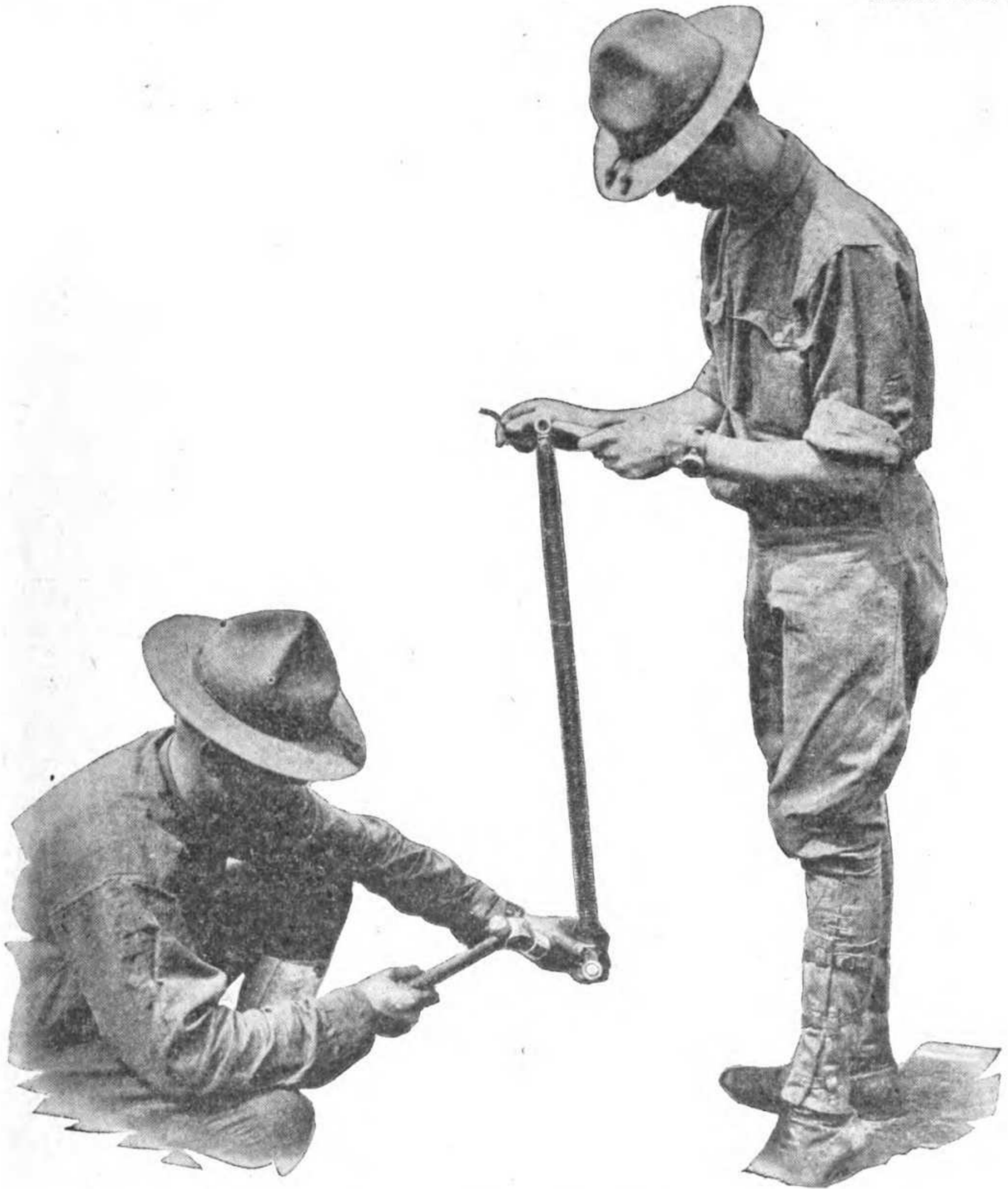
PLUGGING DAMAGED RADIATOR SECTION.
