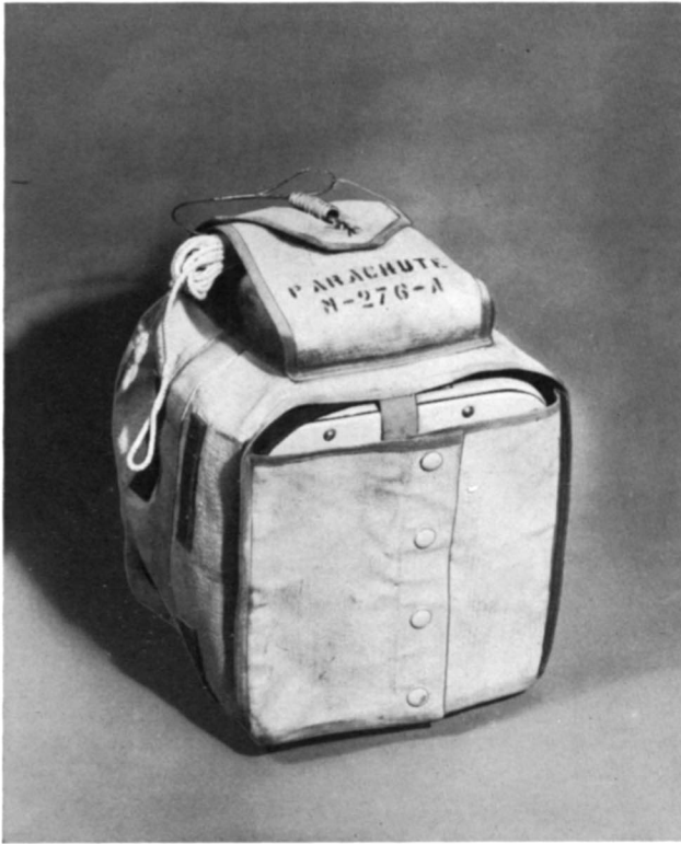
Fig. 7 — Parachute M-276-A, Packed and with Static Line in place
