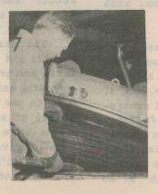
1. A few years ago this tire would have been discarded as worn out. But with present methods of tire reconditioning it can be restored to useful life through recapping.
