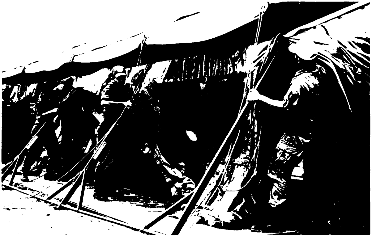
Figure 42. Push up frame, pull in leg
