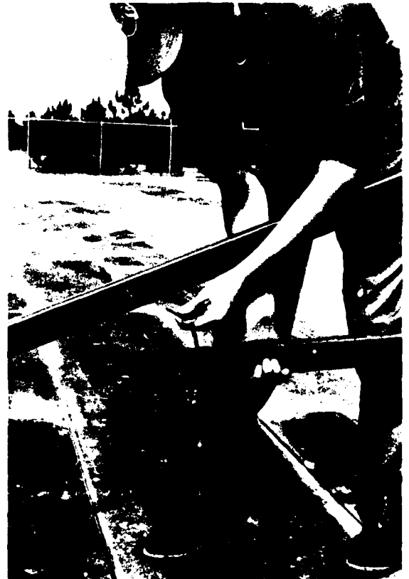
Figure 15. Securing header with locking pin
