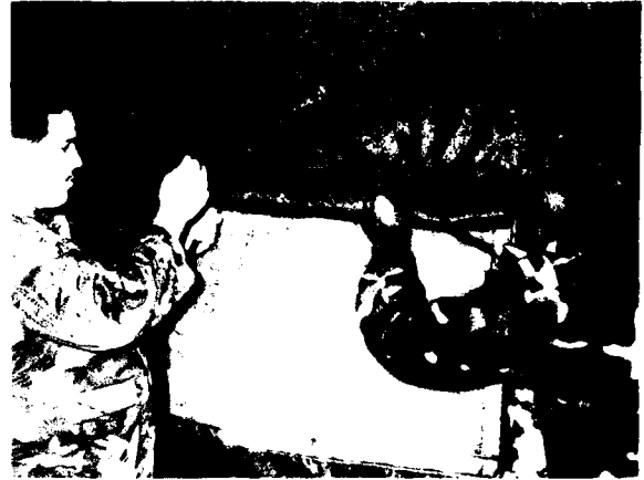
Figure 71. Windows are rolled up towards the inside and tied at the top
