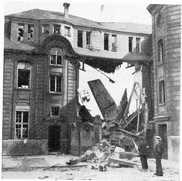
JUST A FEW MOMENTS BEFORE THEY FLED THE CITY, JERRIES BLEW UP THIS LUXEMBOURG TELEPHONE CENTER EARLY IN SEPTEMBER.
