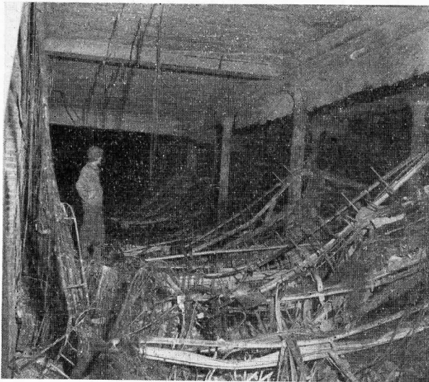
THE MAIN FRAME ROOM OF THE LIEGE TELEPHONE EXCHANGE AFTER IT HAD BEEN BLASTED BY RETREATING NAZIS.
