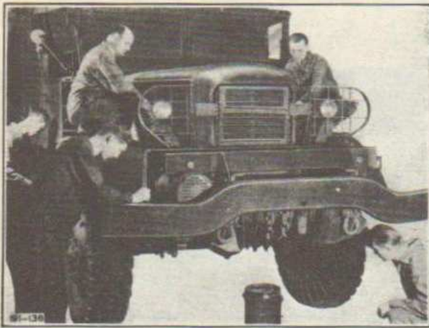
Fig. 25—Five-man Crew Beginning Work of Engine Removal
