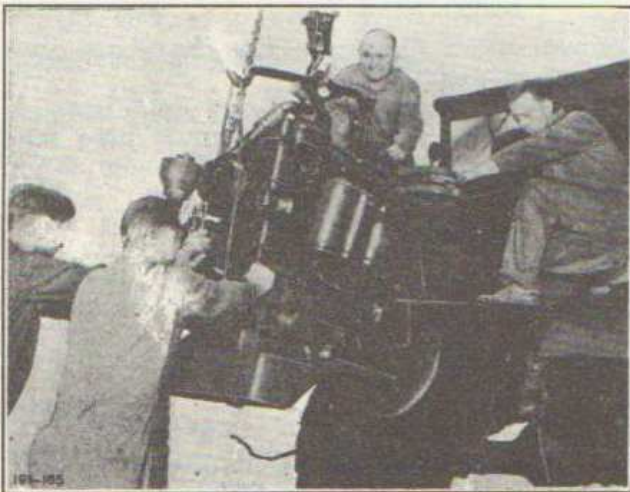
Fig. 137—Placing Engine in Position in Chassis
