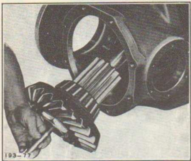
Fig. 45—Installing Spur Pinion Shaft and Bevel Gear Assembly
