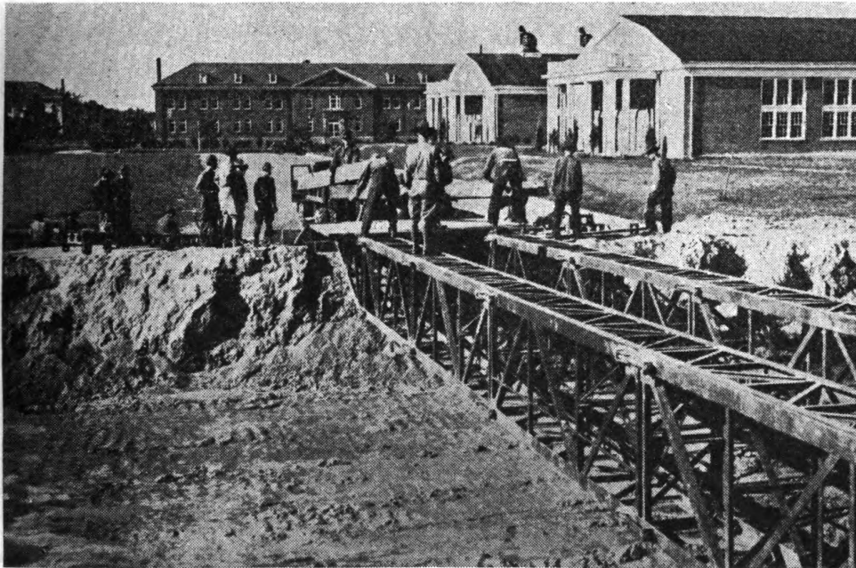
FIGURE 67.—Laying the decking.
