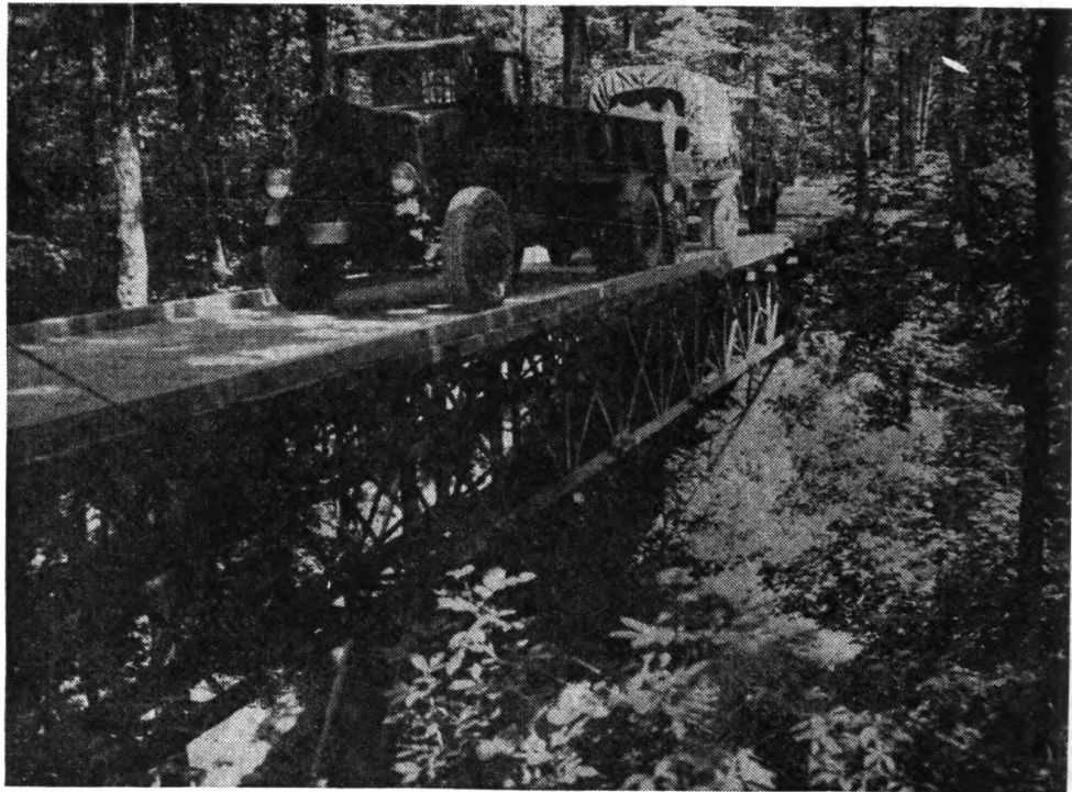
FIGURE 69.—H-20 portable steel bridge.
