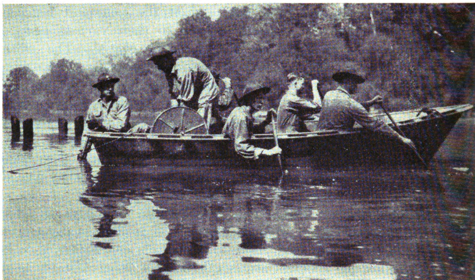
FIGURE 16.—Anchor cable being carried across river in assault boat.
