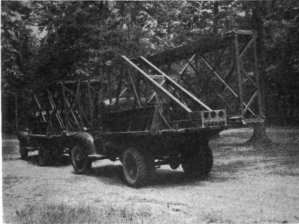
FIGURE 73.—Typical girder loads—1½-ton trucks.
