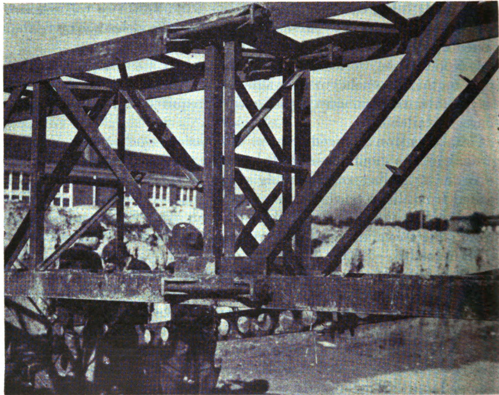
FIGURE 58.—Details of connection between girder sections.
