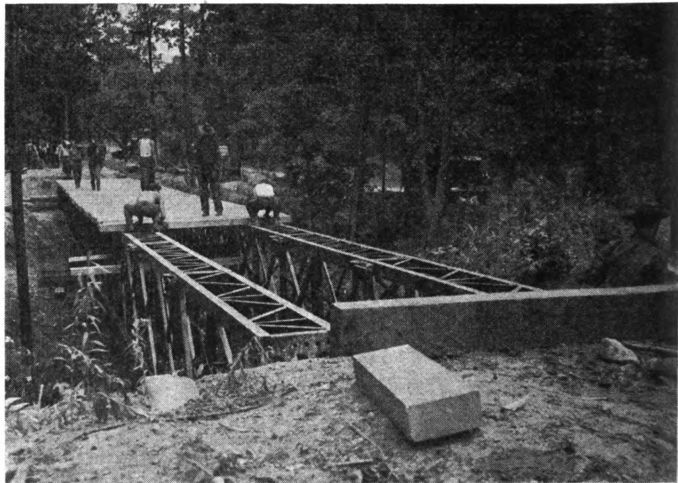
FIGURE 75.—Laying the decking.
