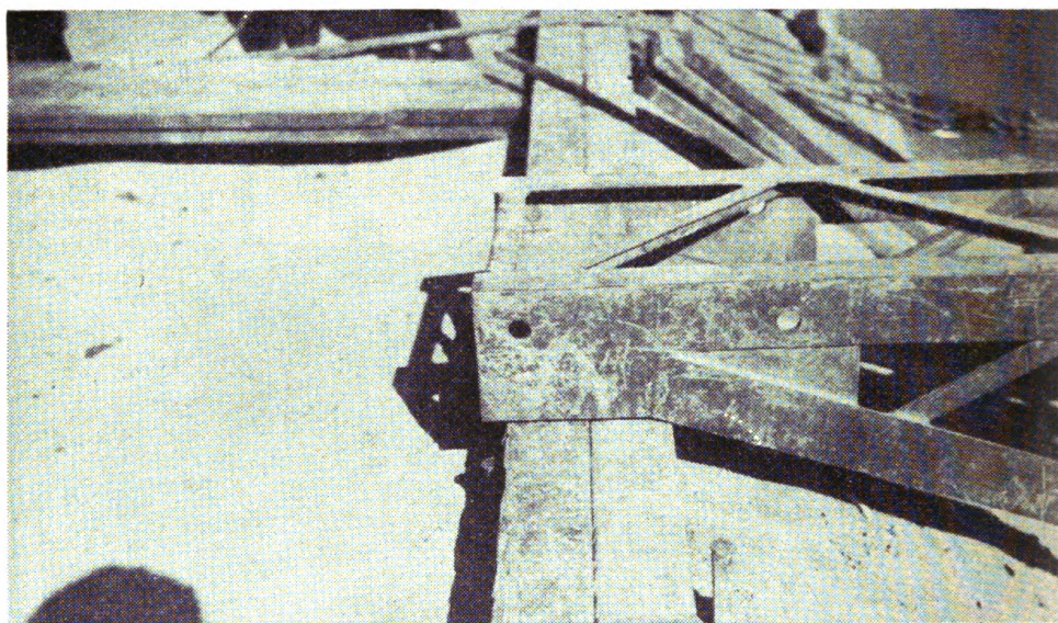
FIGURE 61.—Triangular girder section resting on improvised sill.
