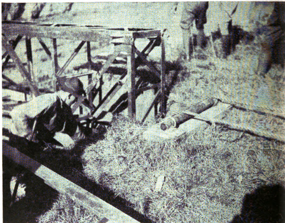
FIGURE 64.—Placing rectangular section on sill (triangular section not used).
