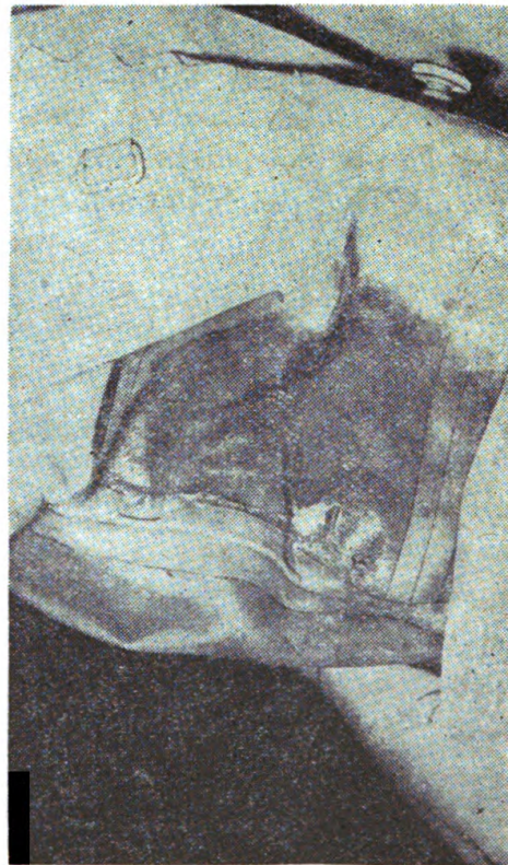
④ Outside patch in place.
