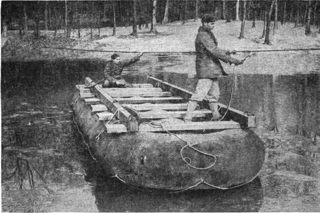
FIGURE 12.—Attaching upstream bridle line to upstream anchor cable.
