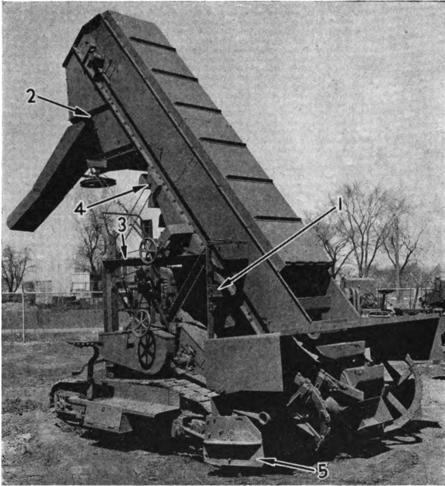
Figure 114. Loader in normal operating position. For ordinary loading operations, Plate 5 is removed from scraper.
