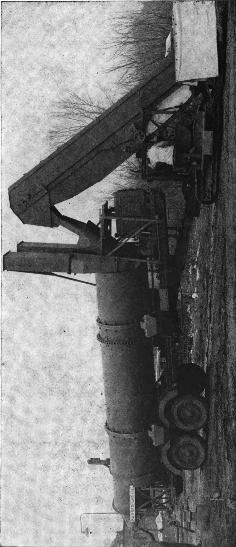
Figure 3. Barber-Greene Paving Loader Being Used in Conjunction with B-G Dual Drum Dryer in Travel Dryer Operation.
