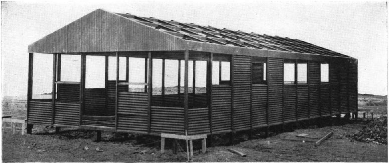
Figure 26. Building end erected and in place.
