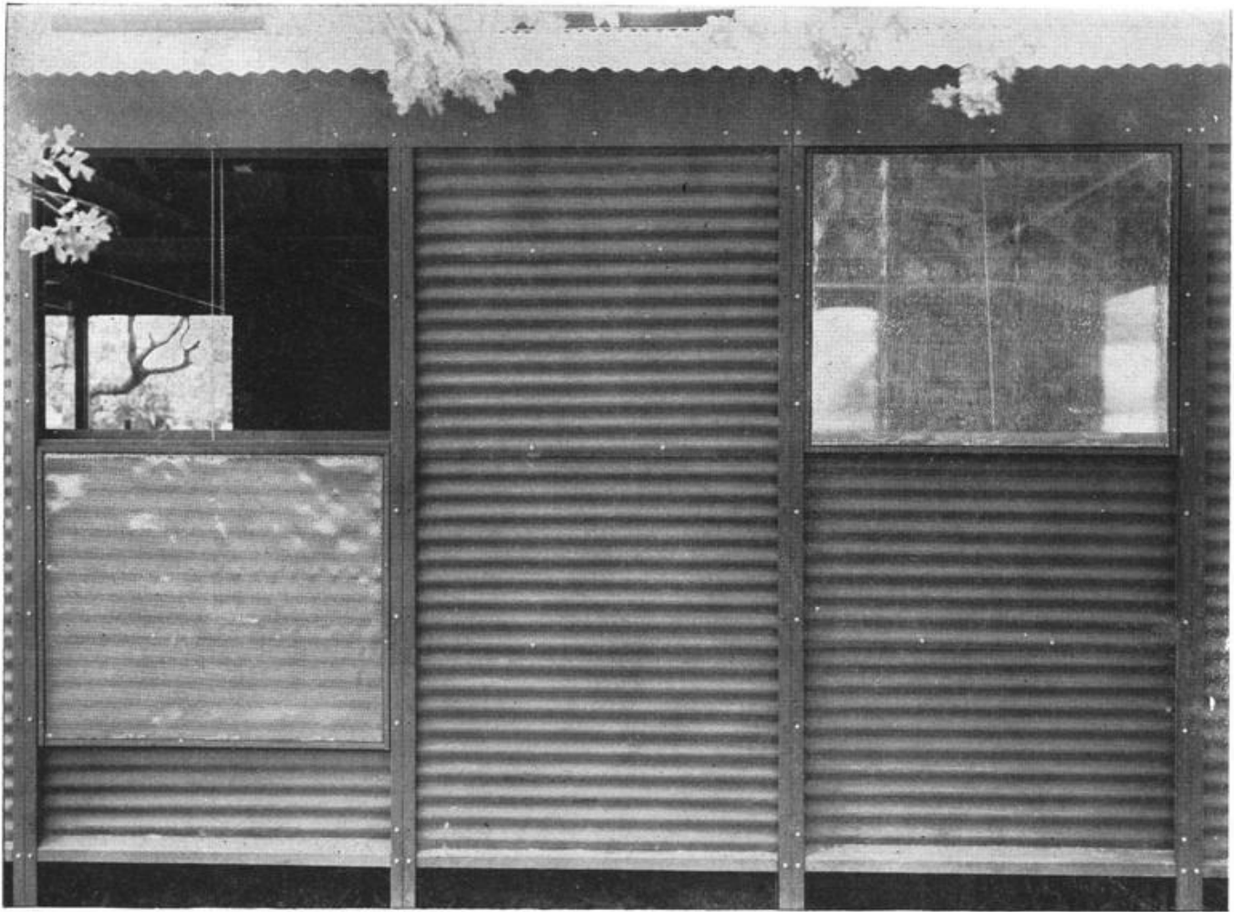
Figure 29. Detail view of side wall panels showing window in place.
