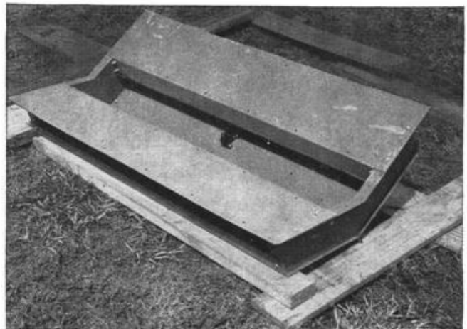
Figure 15. Assembled ridge ventilator showing location of pulley before applying screening.
