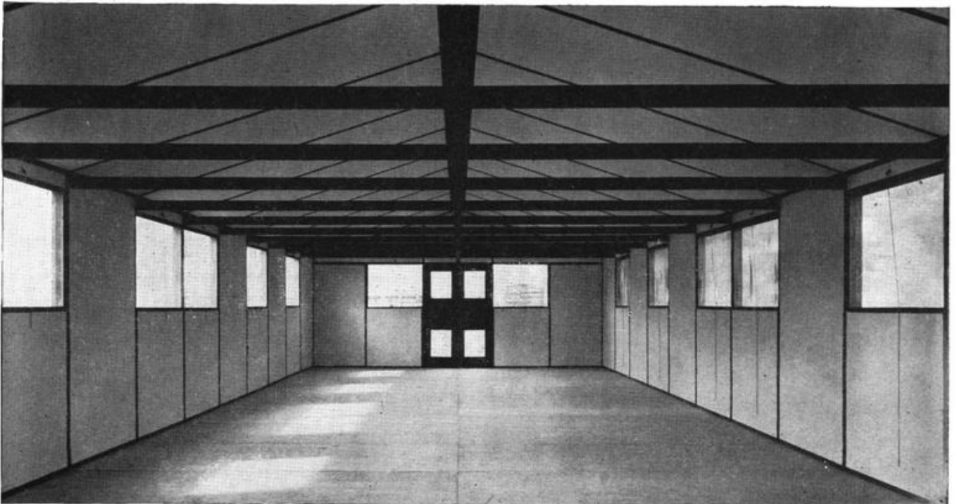
Interior view completed building.
