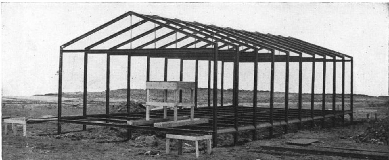
Figure 19. All building ribs erected and showing platform from crating material.
