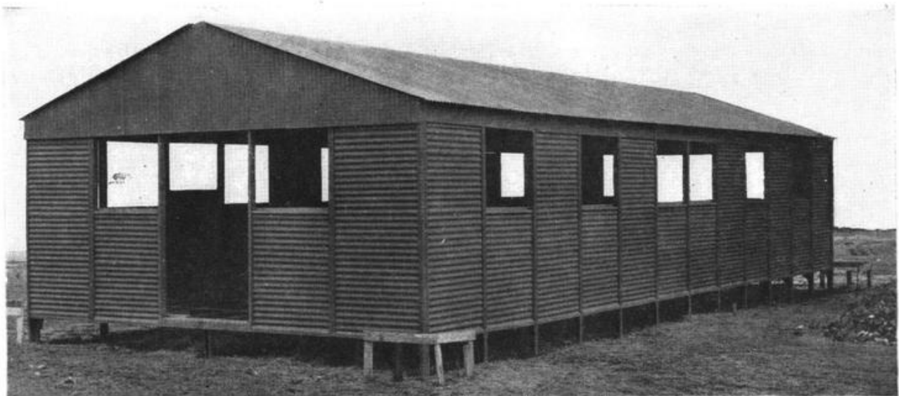
Figure 27. Roofing panels applied.
