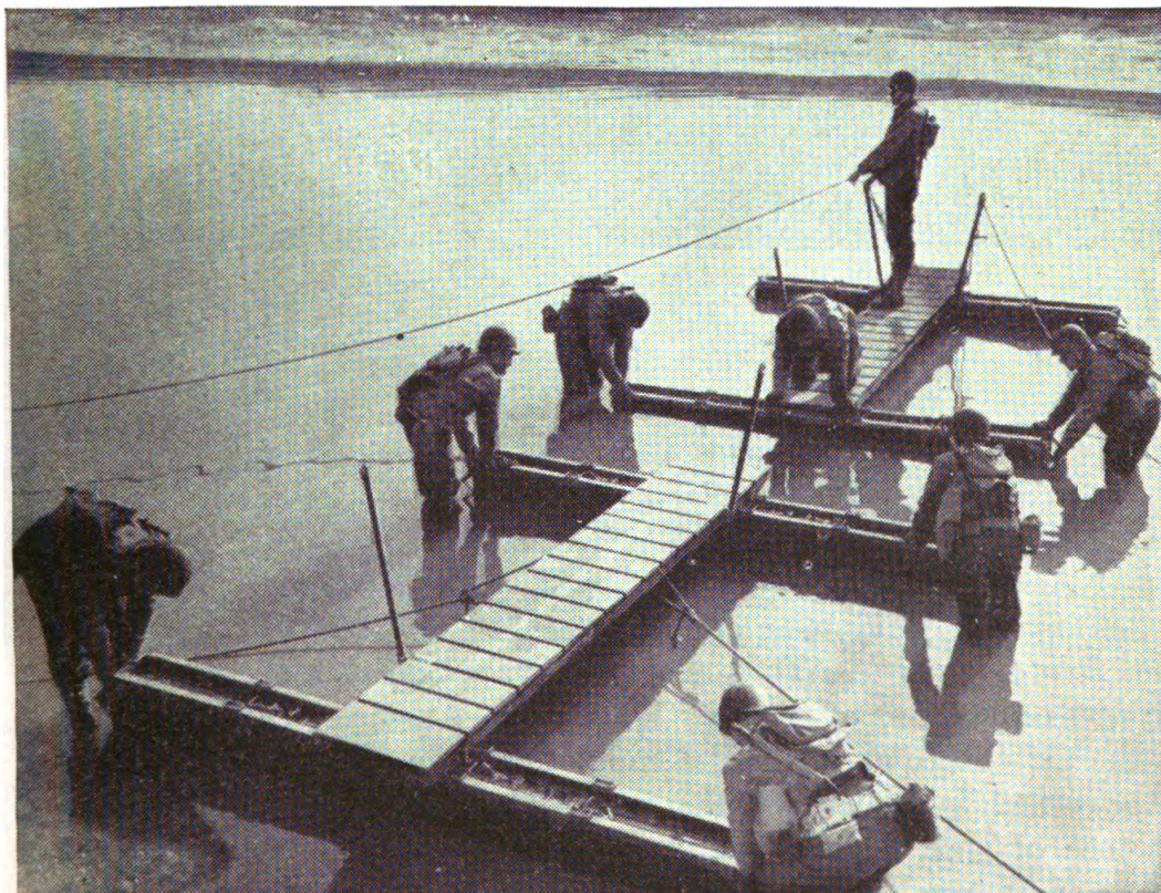
FIGURE 45.—Bay with guy lines attached being connected to bridge.
