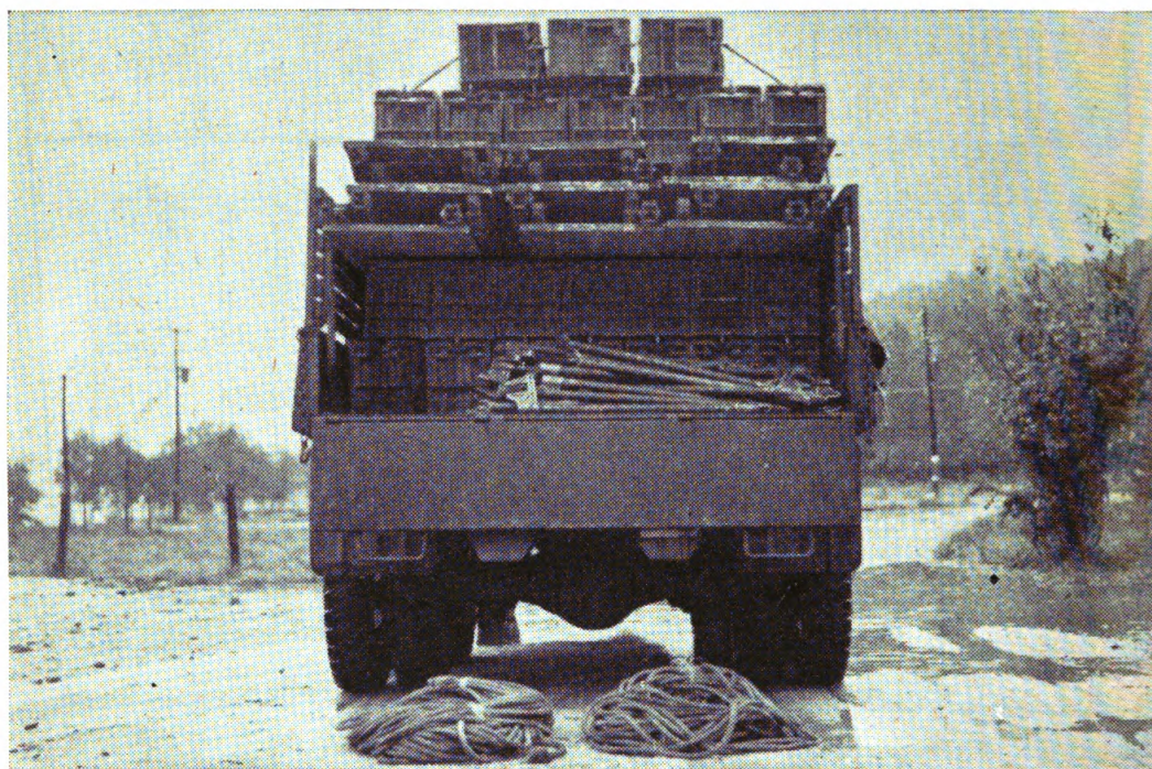
FIGURE 51.—Typical loading of 2½-ton truck.
