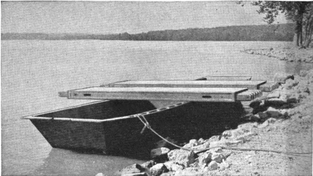
FIGURE 14.—First pair of treadways placed on first assault boat ponton.
