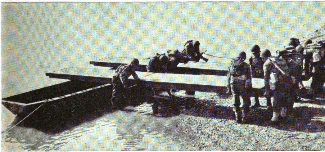
FIGURE 15.—Connecting second pair of treadways.
