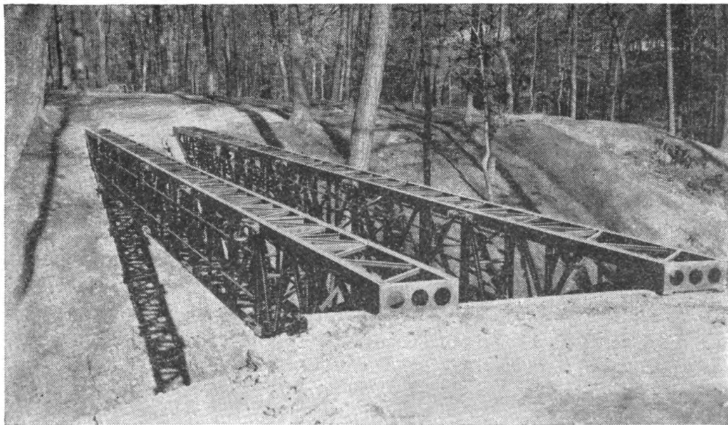
FIGURE 3.—Trusses in place across gap.
