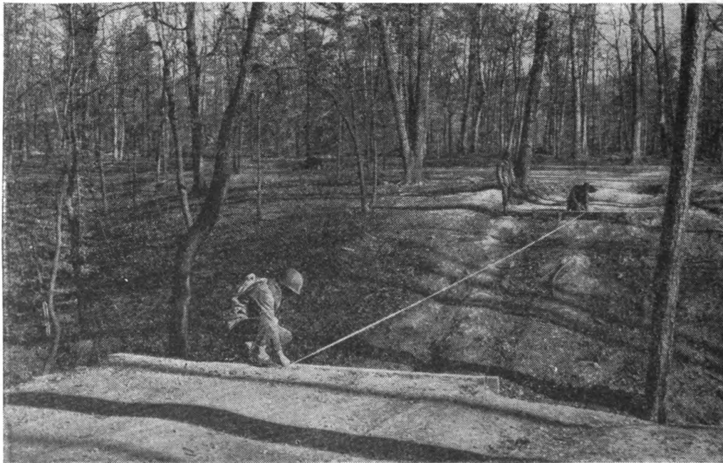
FIGURE 29.—Distance between abutment sills being checked.
