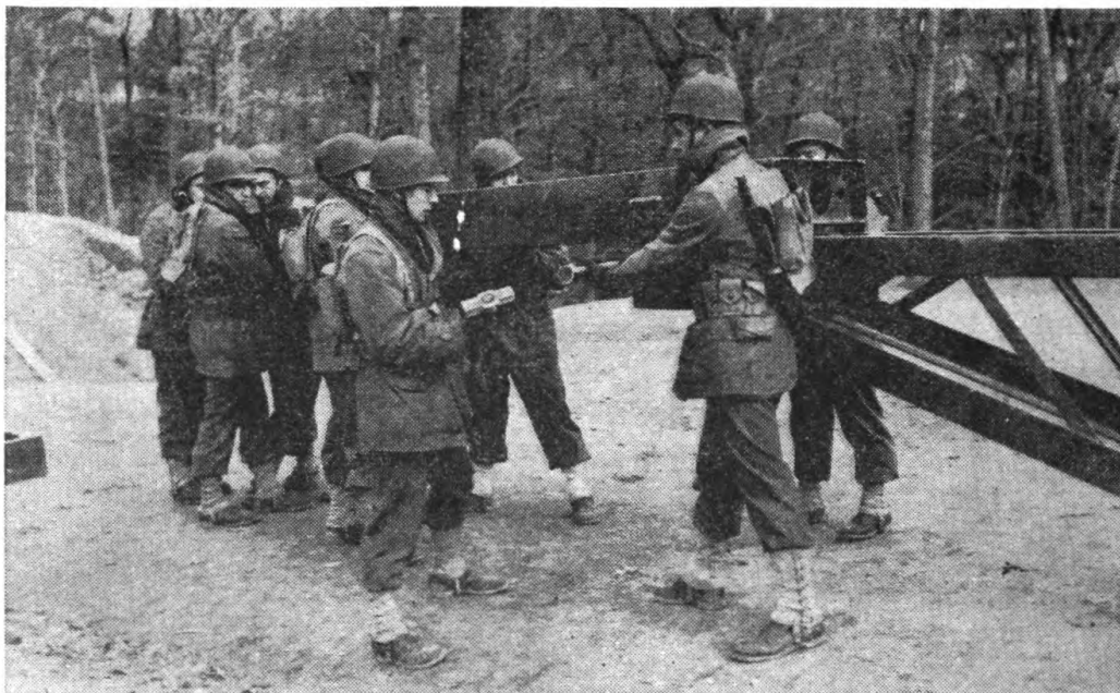
FIGURE 20.—Rear section of launching nose being attached to end section.
