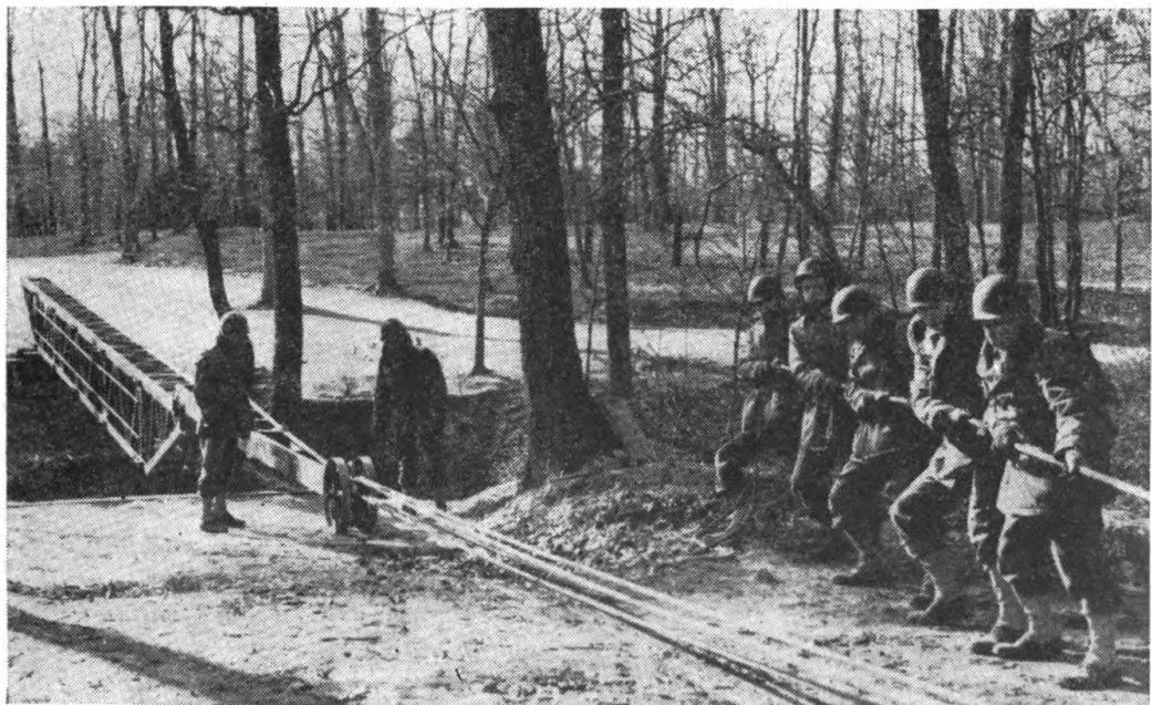
FIGURE 35.—Launching nose being hauled upon a far bank.
