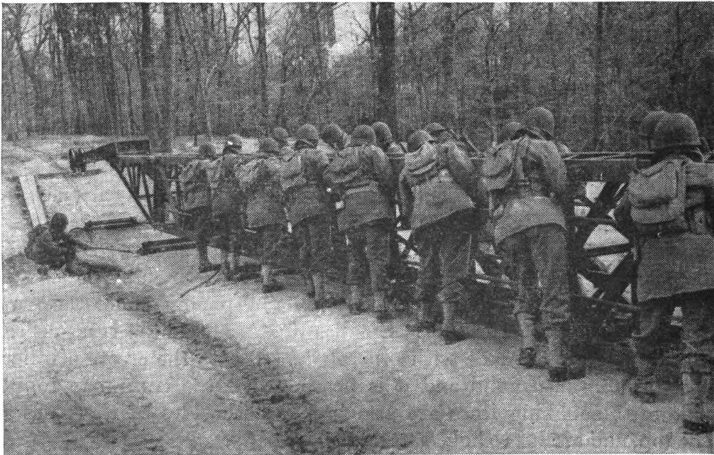
FIGURE 31.—Truss being pushed out on erection rollers.
