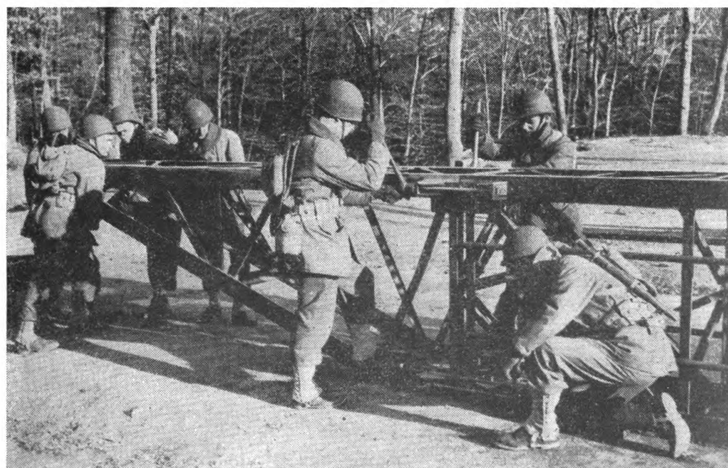
FIGURE 19.—End and intermediate sections being bolted together.
