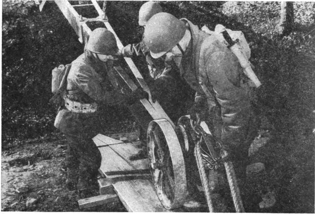
FIGURE 34.—Details of block and tackle connected to launching nose.
