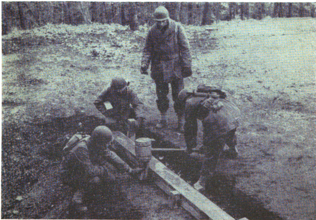
FIGURE 27.—Abutment sill being secured in place.
