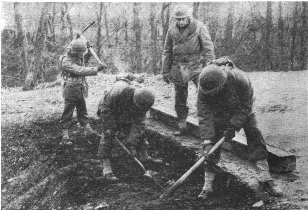
FIGURE 25.—Cutting down bank for abutment sill.
