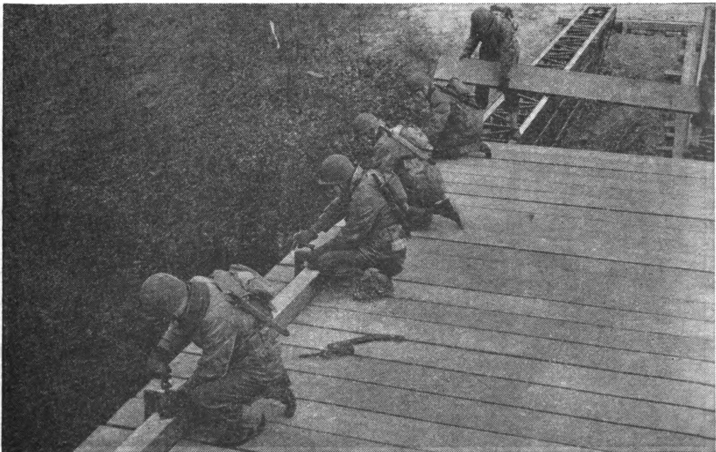
FIGURE 41.—Attaching siderails.
