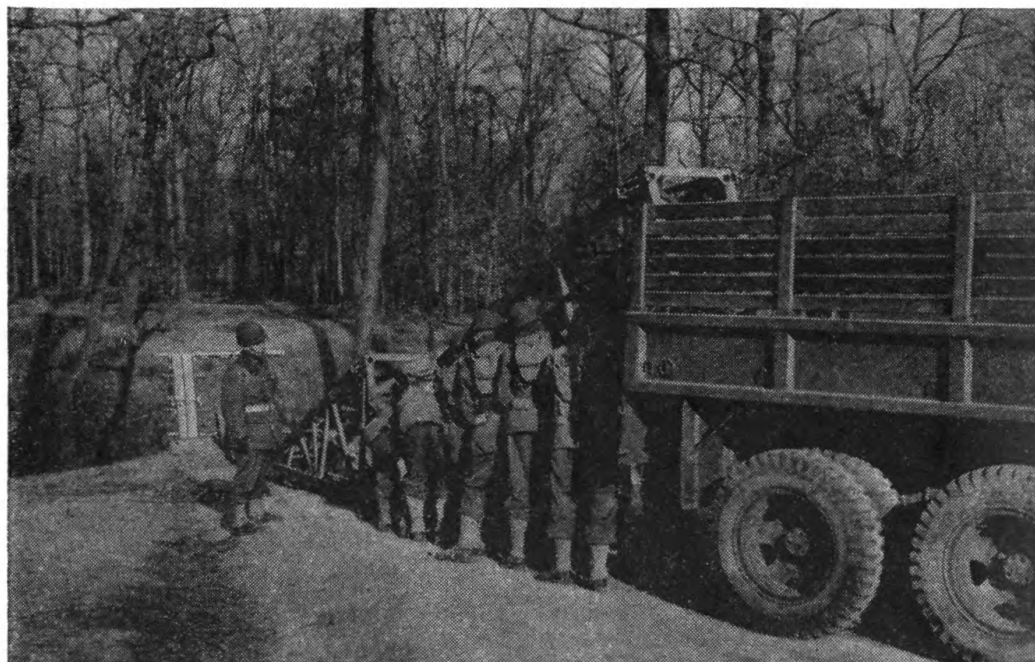
FIGURE 18.—Intermediate section being unloaded from truck.
