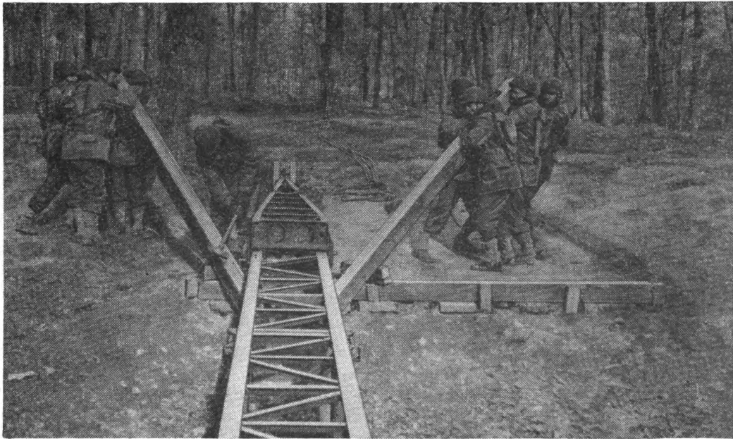
FIGURE 37.—Raising truss section in order to disengage launching nose.
