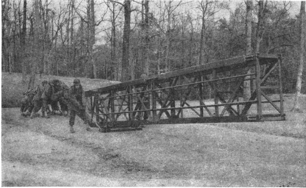
FIGURE 22.—Erection roller being inserted beneath truss.
