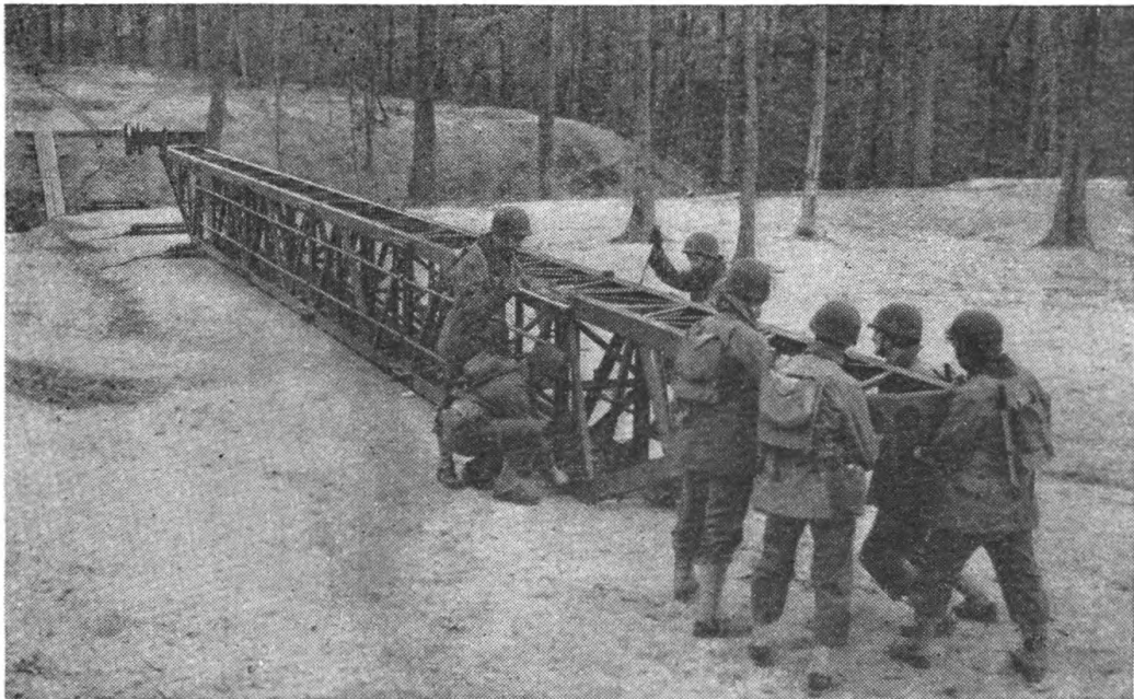
FIGURE 23.—Last section of truss being bolted.
