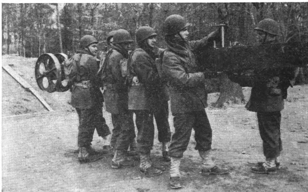
FIGURE 21.—Front section of launching nose being attached to rear section.
