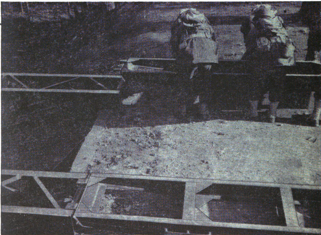
FIGURE 39.—Second abutment ramp being placed.
