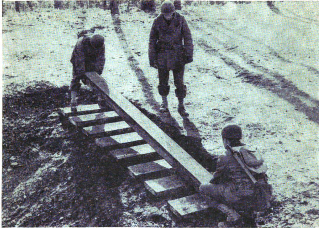
FIGURE 26.—Placing abutment sill on footings.
