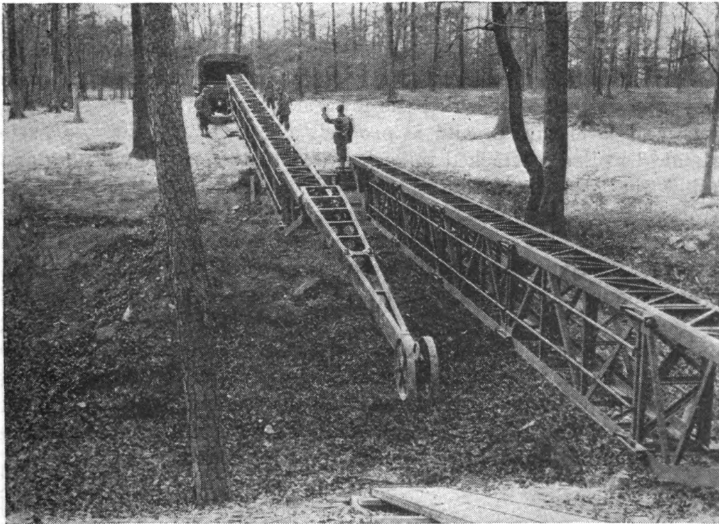
FIGURE 45.—Truss being hauled out by truck.
