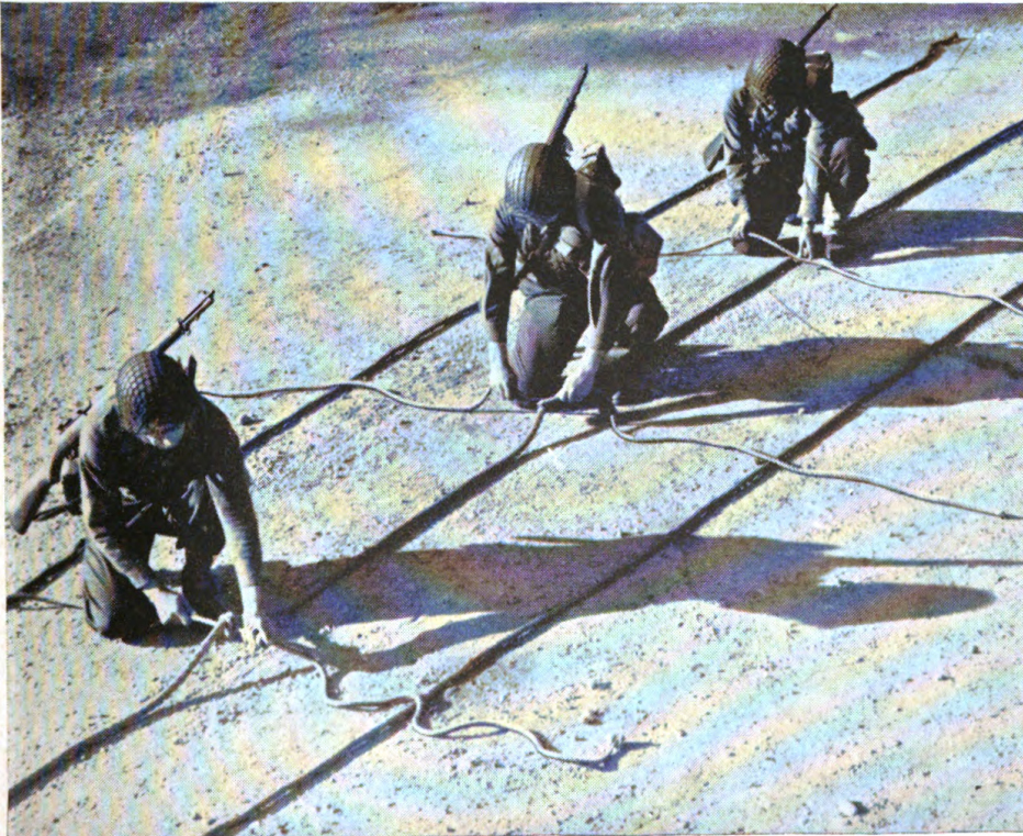
FIGURE 42. Erection of three-rope bridge. (1) Ropes are laid out on ground near site. (2) Suspenders are tied to tread rope.
