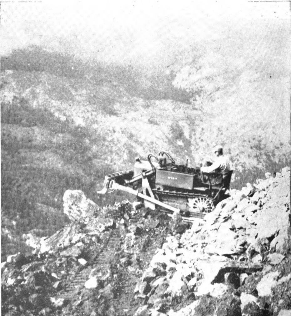
FIGURE 34. Trail tractor. Used to clear and construct trails and light-equipment roads.
