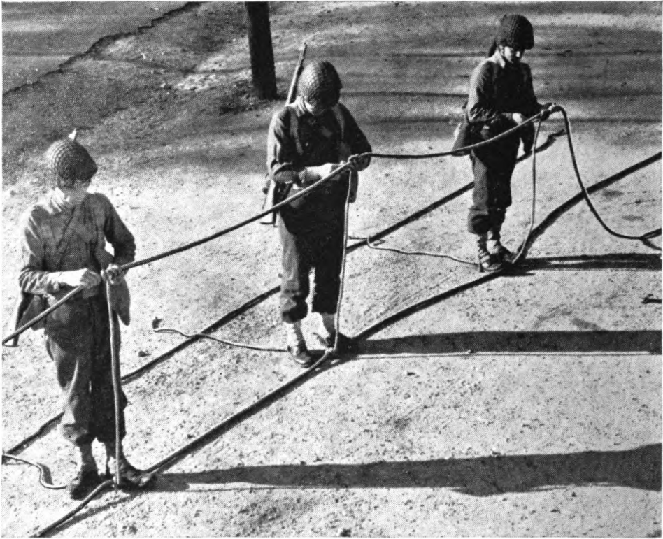
FIGURE 42. Erection of three-rope bridge. (3) Suspenders are tied to hand rope. Note that hand rope is elbow-high. (4) Assembled bridge is carried into position.
