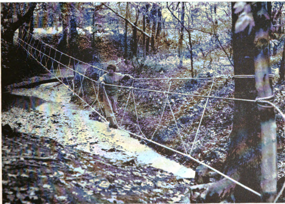
FIGURE 41. Three-rope bridge. An expedient used to cross foot troops.
