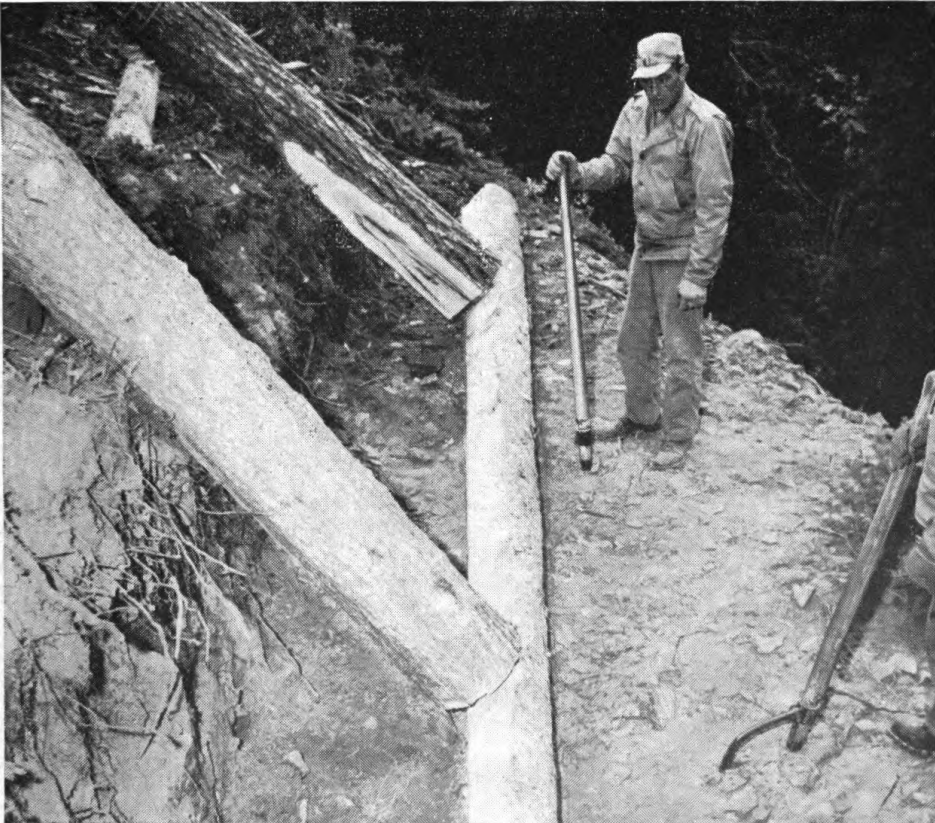
FIGURE 23. Tower sill on rock foundation. Sill foundation is levelled. Footings may be used to spread loads.
