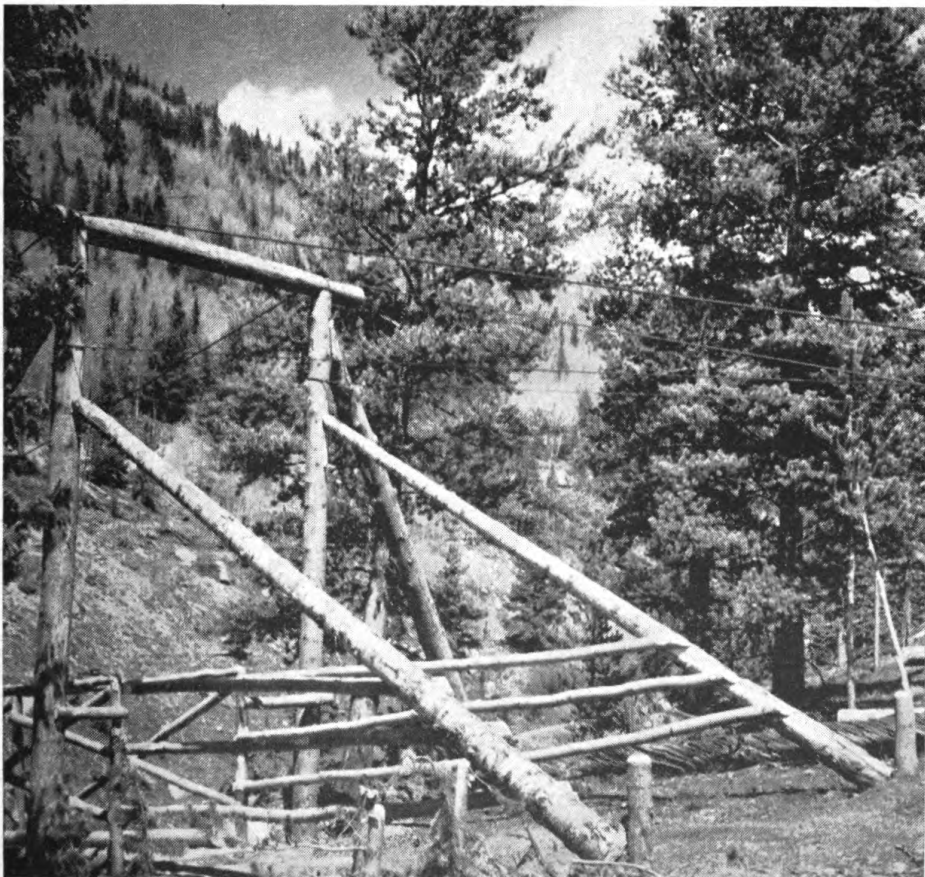
FIGURE 31. Approach siderails. Used to guide men and animals from approach trail to bridge.
