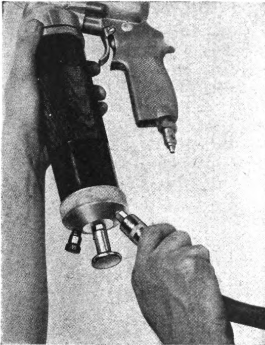
Figure 63 Applying Air Pressure to Primer Valve
