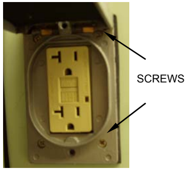
Figure 10. Receptacle Cover Screws.
