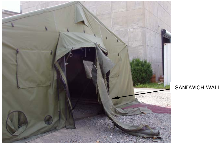
Figure 10. Partially Attached Sandwich Wall
