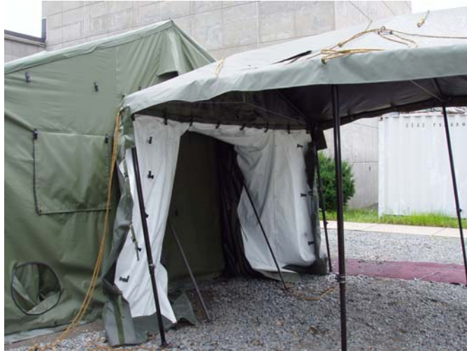
Figure 14. Second Vestibule Frame, Attached.
