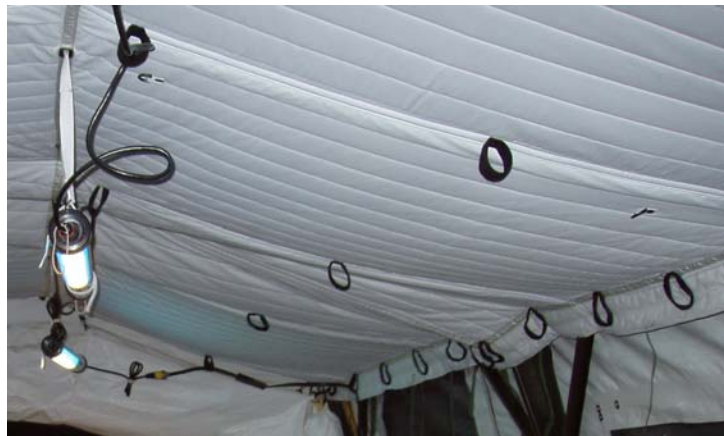
Figure 60. Cable Management System on the Roof Cap Liner.
