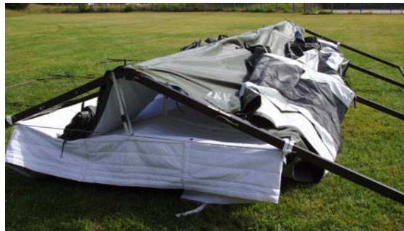
Figure 21. Draping Fabric Over Frame.
