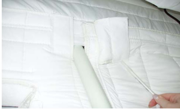
Figure 43. Feeding Power Panel Stand Through Wall Liner Notch.
