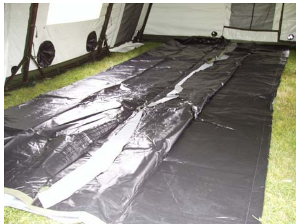
Figure 41. Unrolling Fabric Floor Inside Tent.
