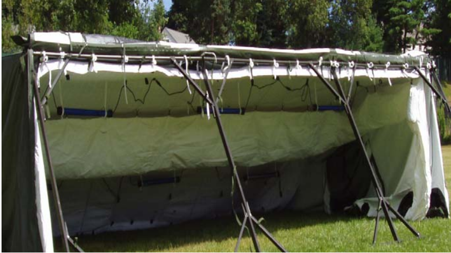
Figure 34. Attaching Roof Cap Liner to Tent Frame at Eave.
