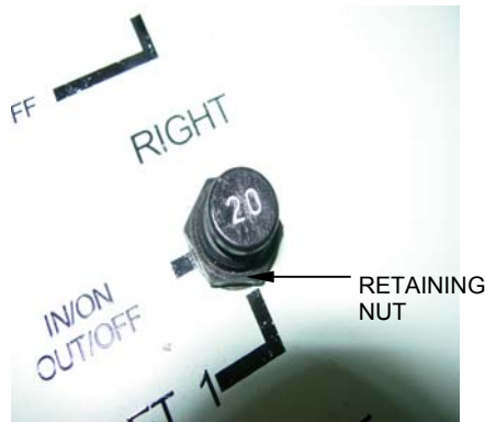
Figure 3. Circuit Breaker Retaining Nut.
