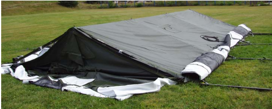
Figure 28. After Attaching Endwall Sections.
