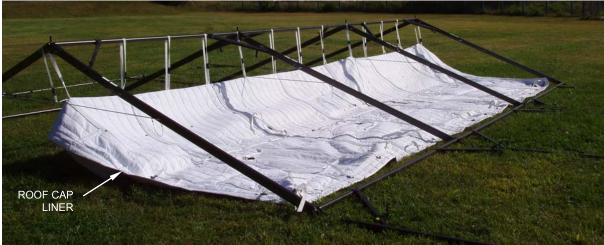
Figure 16. Insulated Roof Cap Liner.
