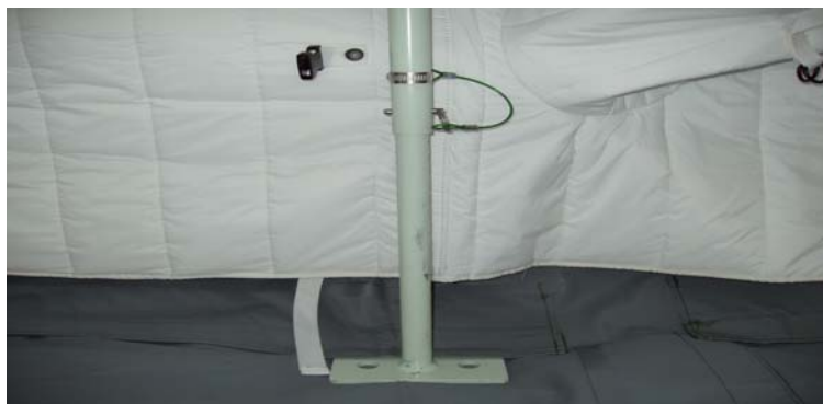
Figure 45. Locking Power Panel Stand In Place.
