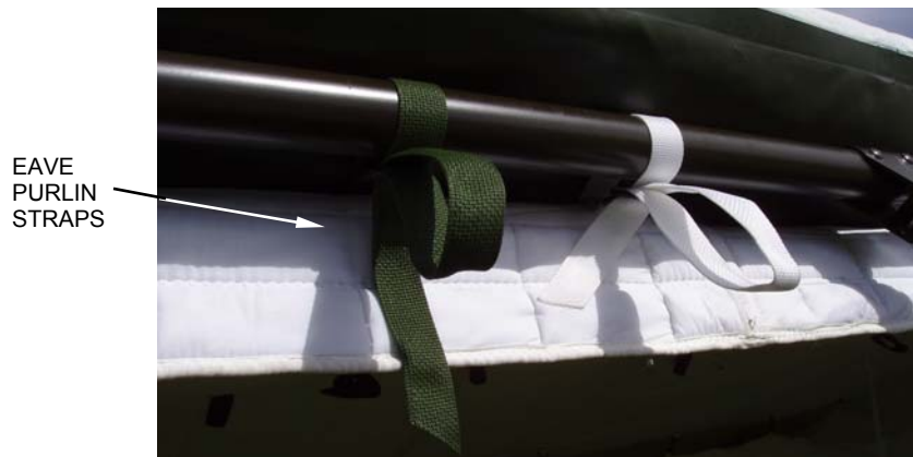
Figure 33. Securing Eave Purlin Straps.
