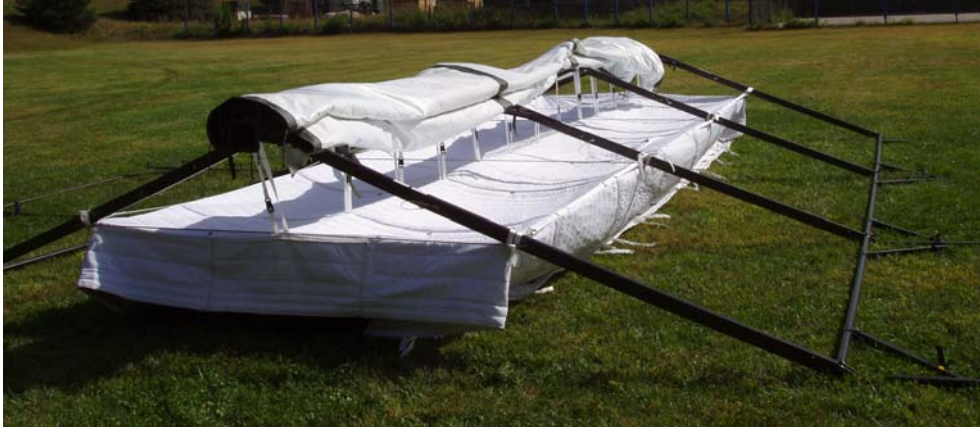
Figure 20. Placing Fabric On Tent Frame Ridge.
