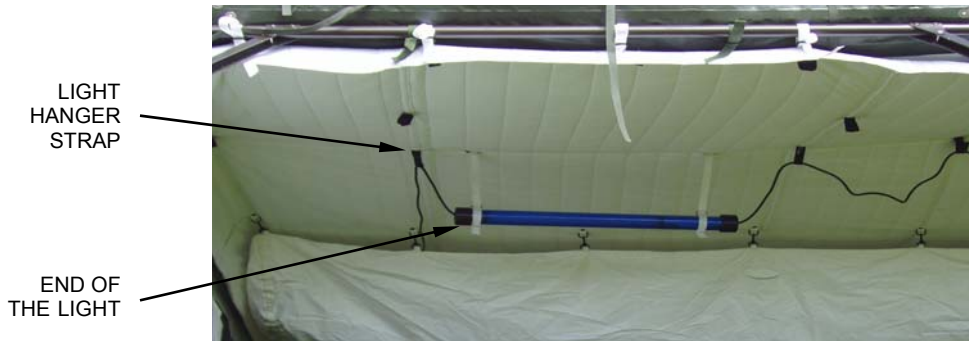
Figure 35. Installing Light Assemblies.
