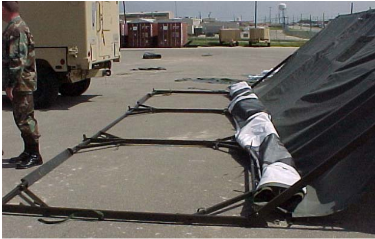
Figure 27. Fabric Section Rolled to Eave.
