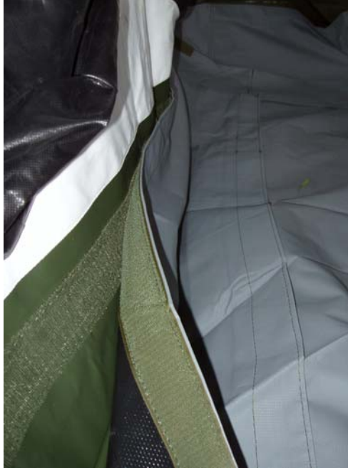
Figure 42. Mating Hook and Pile Fastener and Tape on the Side and End Walls.
