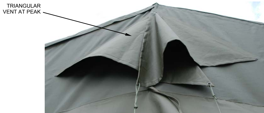
Figure 47. Roof Vent Location.
