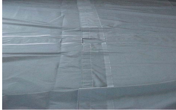
Figure 56. Cable Management System in the Floor in the Closed Position.
