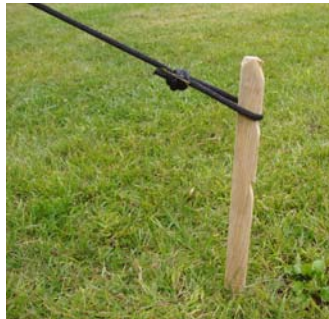
Figure 39. Securing High Wind Lines.
