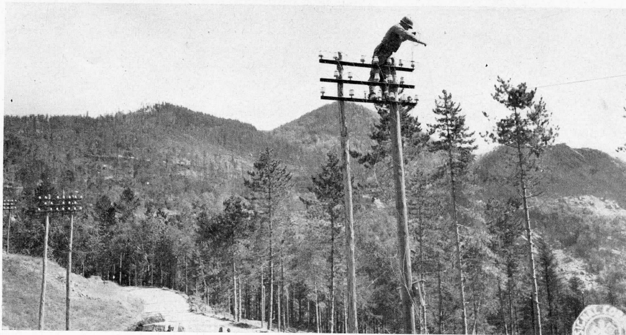
NEAR FIRENZUOLA IN ITALY A SIGNAL CORPS SOLDIER STRINGS WIRE ON AN ITALIAN H-FIXTURE. THE MOUNTAINOUS BACKGROUND INDICATES THE TYPE OF TERRAIN IN WHICH THE BATTLE AGAINST THE GOTHIC LINE WAS FOUGHT.
