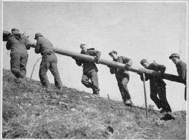
A CREW MANHANDLES A POLE INTO THE PROPER POSITION
