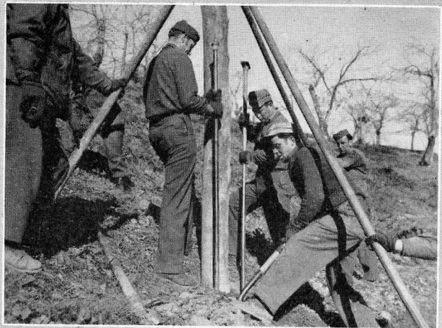
... MEN FILL THE HOLE AND TAMP DOWN THE EARTH
