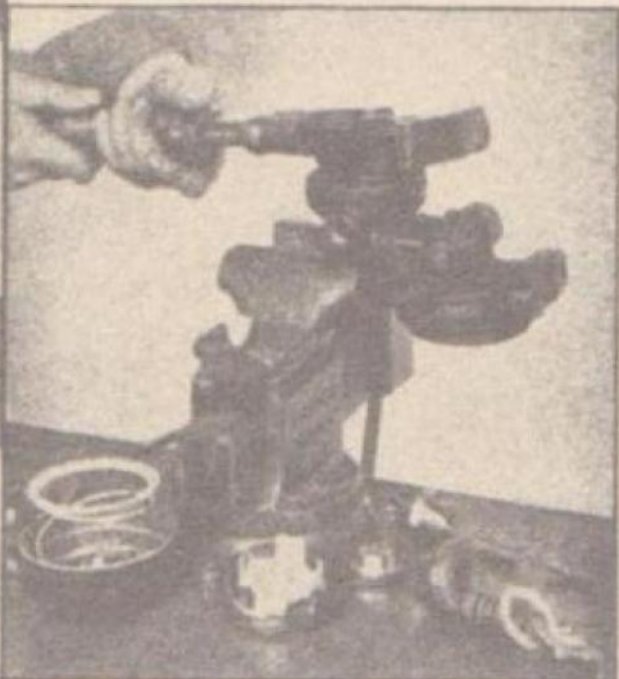
FIGURE G. REMOVING DIAPHRAGM COVER BODY
