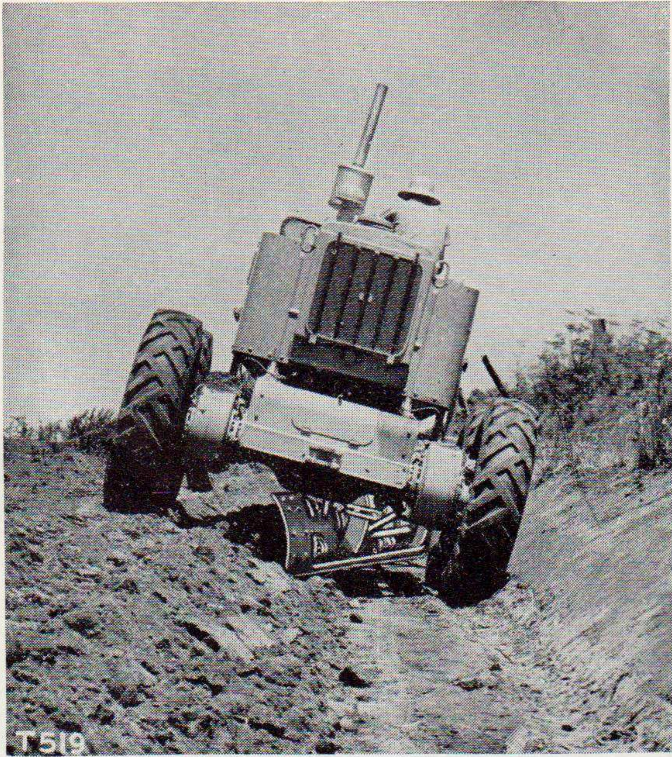
Figure 41. Cutting the flat bottom.
