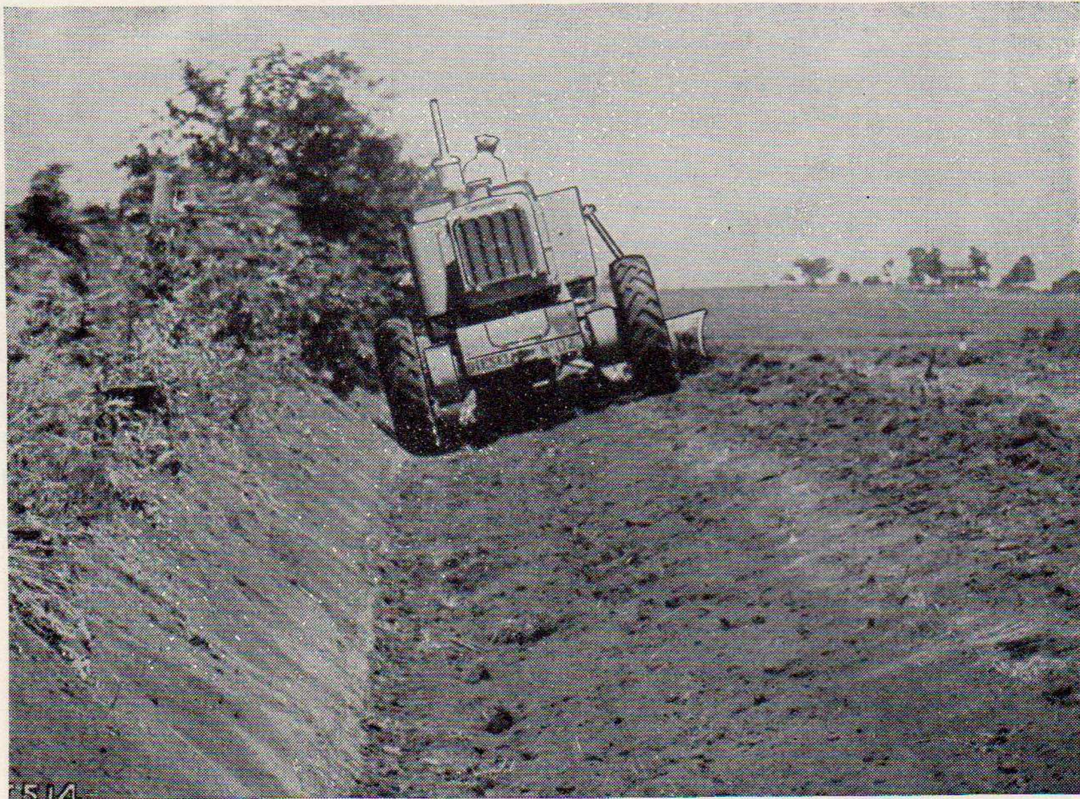
Figure 39. Cutting the inside slope.
