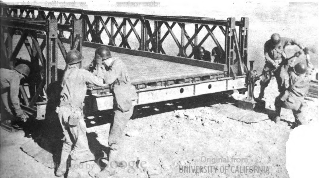
Figure 55.—Jacking up end of bridge before removal of rocking rollers.
