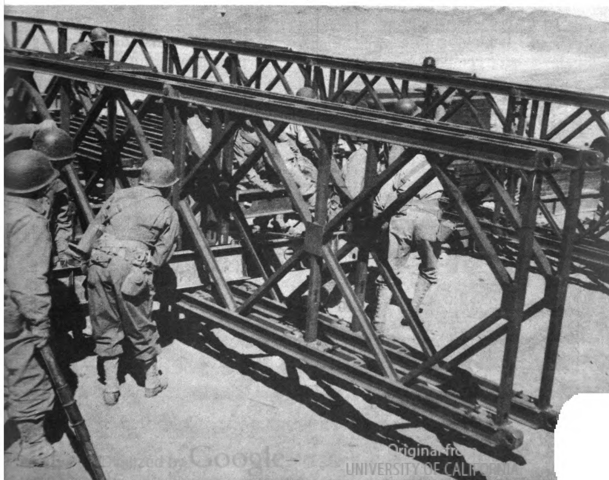
Figure 33.—Transom detail installing panel in place.
