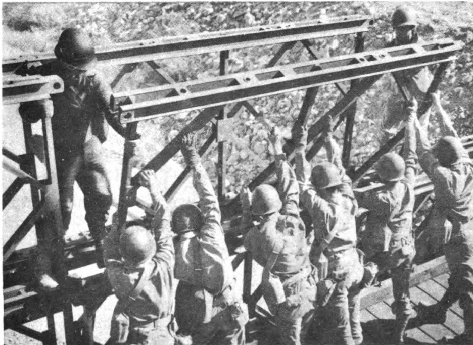
Figure 63.—Placing second-story panel.
