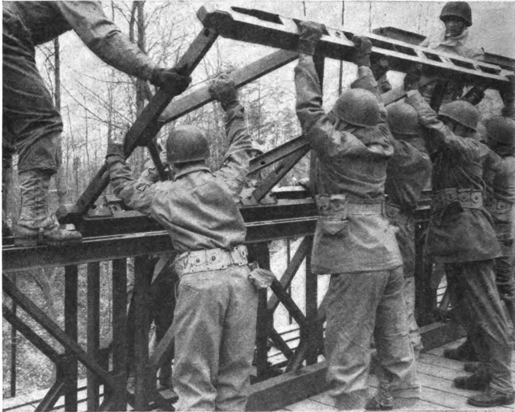
Figure 65.9.—Placing outer-truss second-story panel for converting double-single to double-double bridge.
