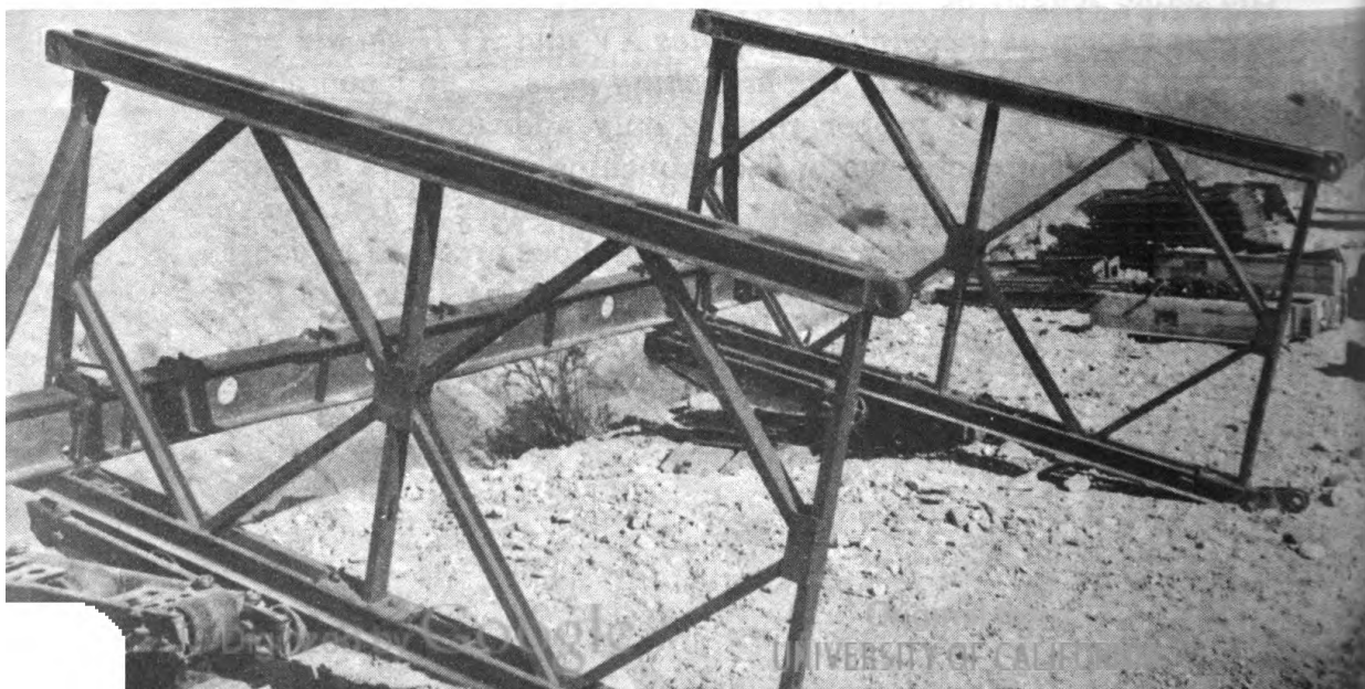
Figure 43.—First bay of launching nose.
