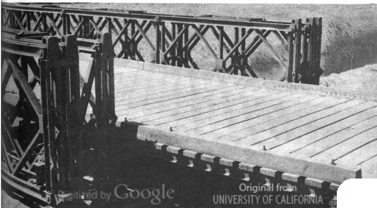
Figure 59.—Single-bay ramp completely decked.
