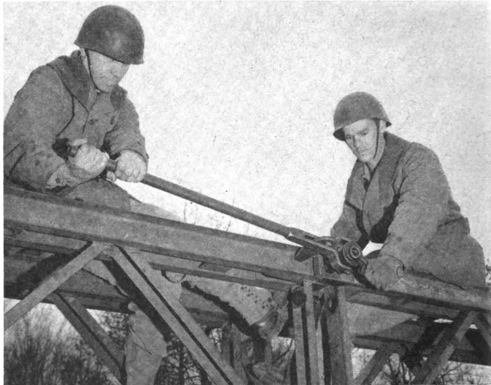
Figure 65.16.—Using pin extractor in dismantling bridge.
