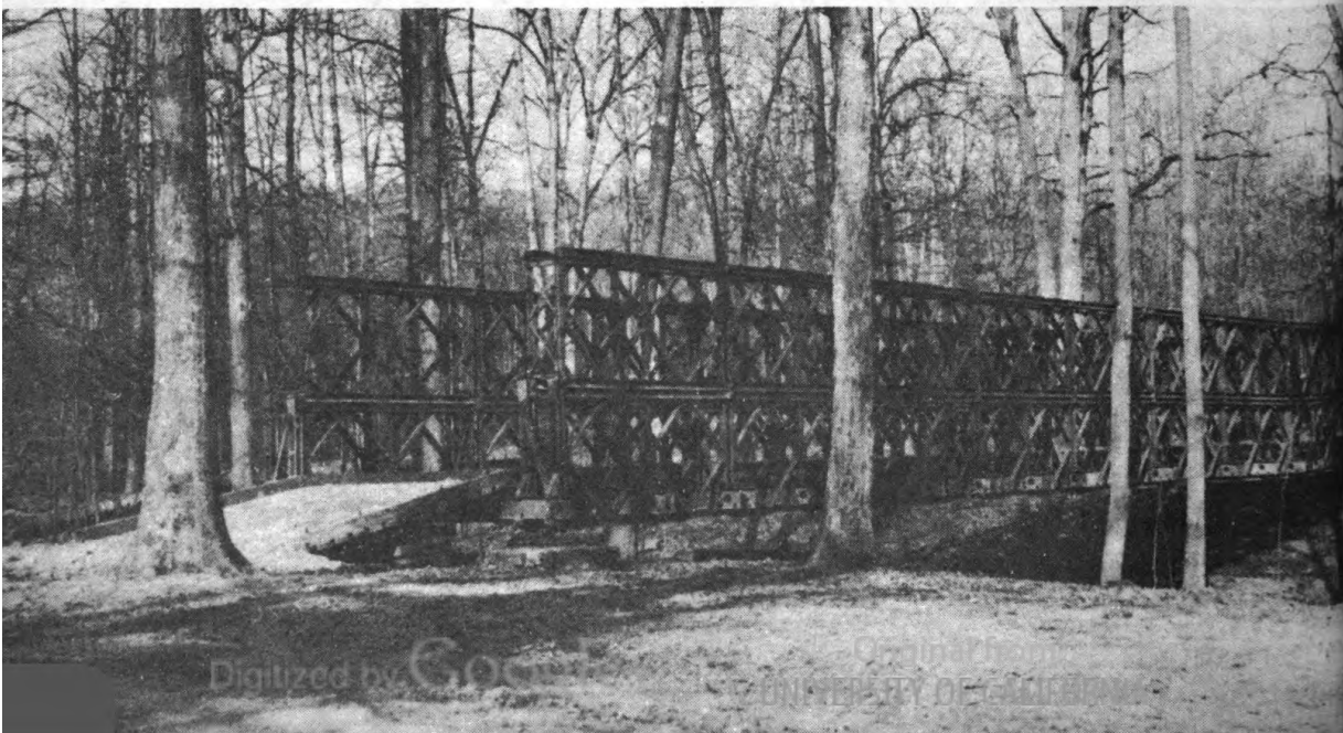
Figure 2.—Double-double bridge.
