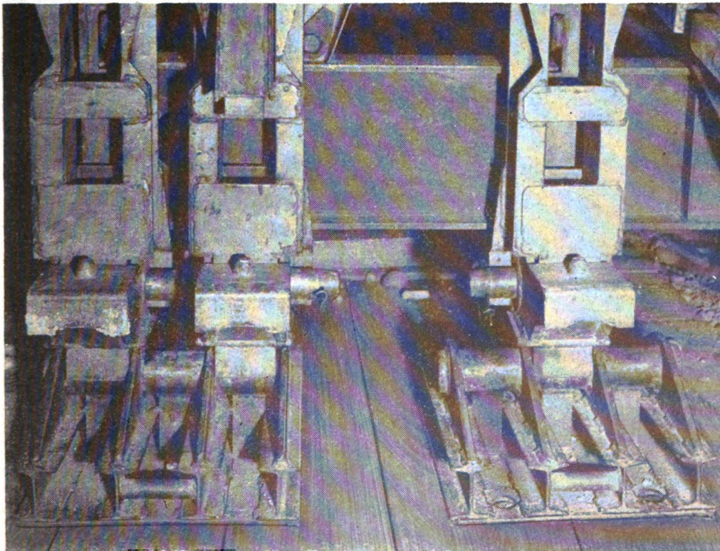
Figure 65.6.—Position of bearings in triple-truss construction.
