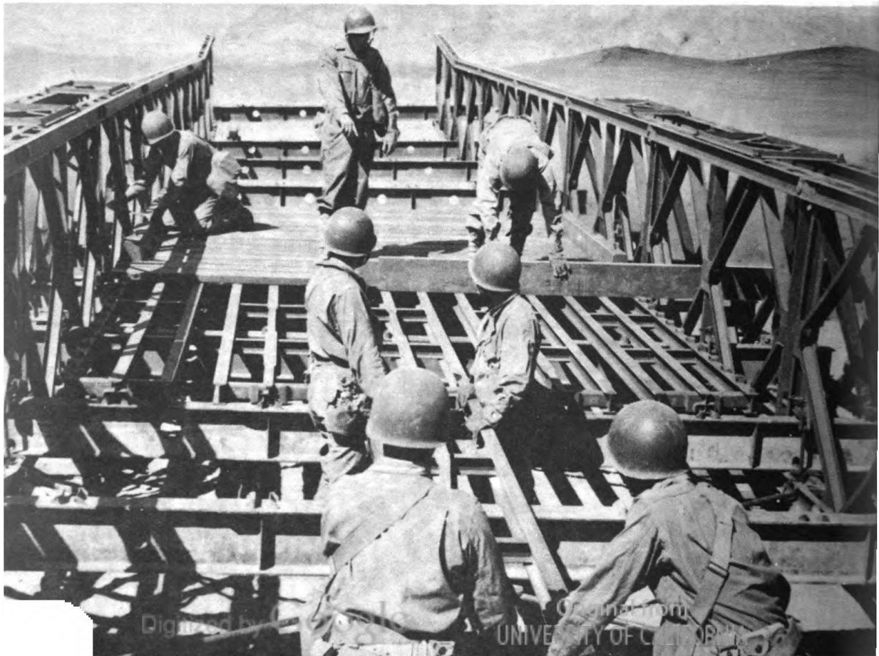
Figure 35.—Decking detail laying stringers, chess, and ribbands.
