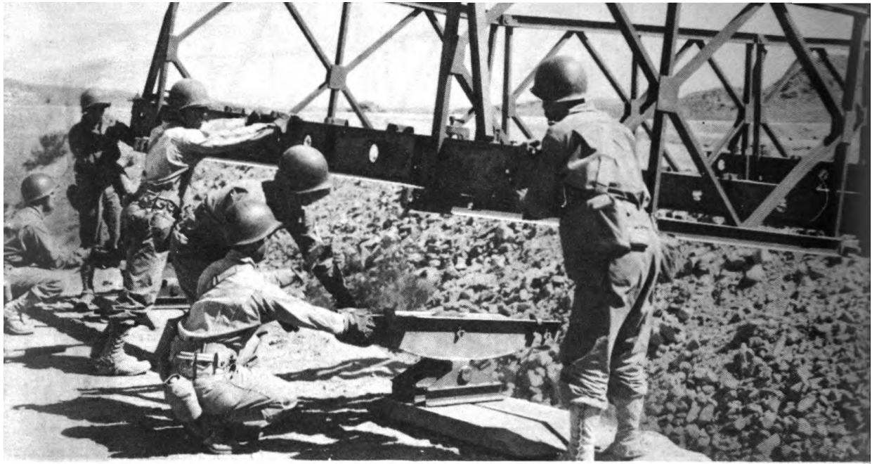
Figure 52.—Guiding launching nose onto rocking rollers.
