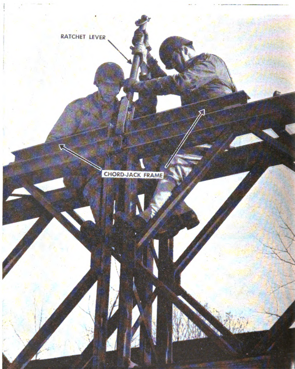
Figure 65.12.—Using chord jack to spread second-story panels of double-double bridge.
