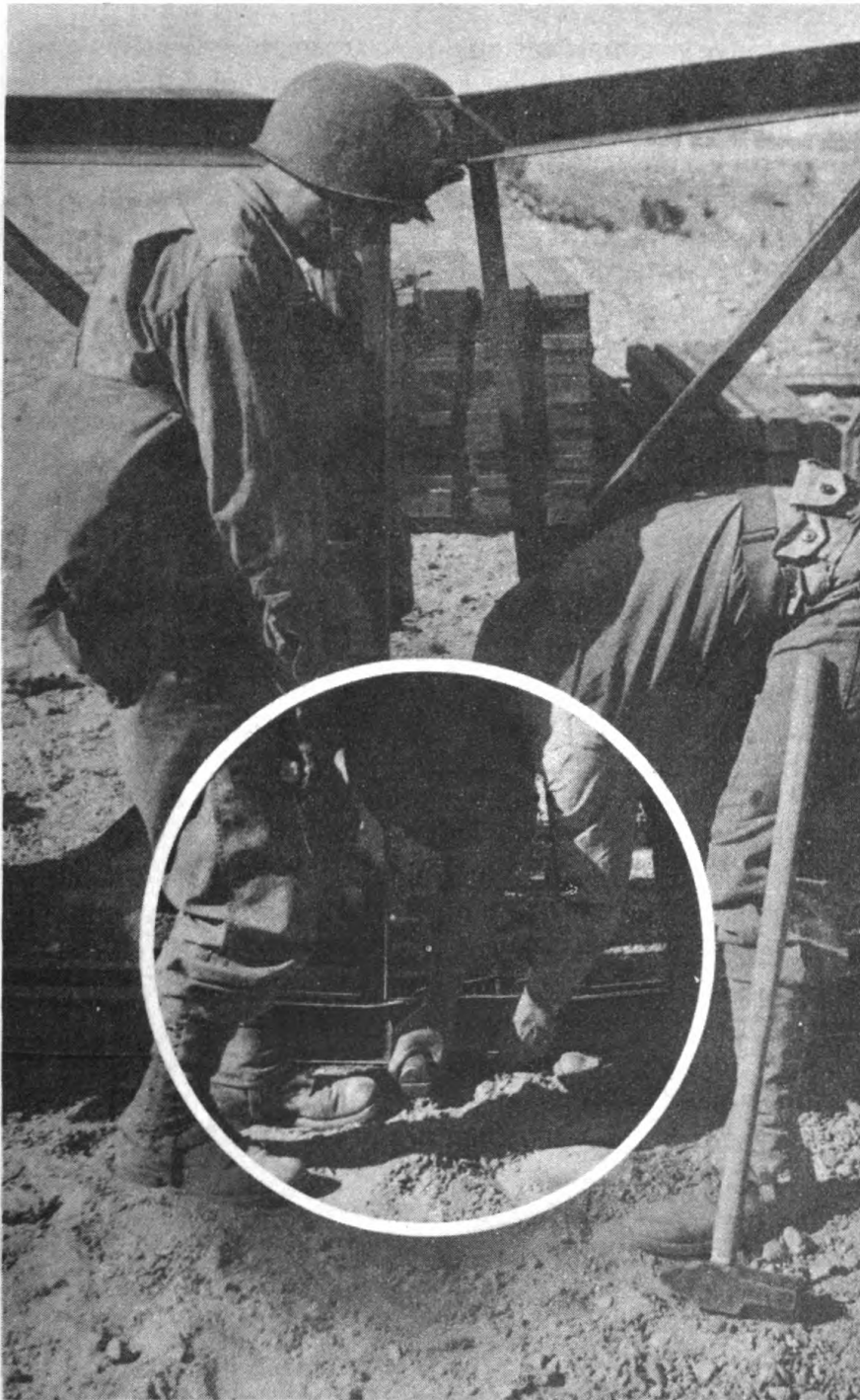
Figure 46.—Inserting panel pin to connect panel in launching nose to launching-nose links.
