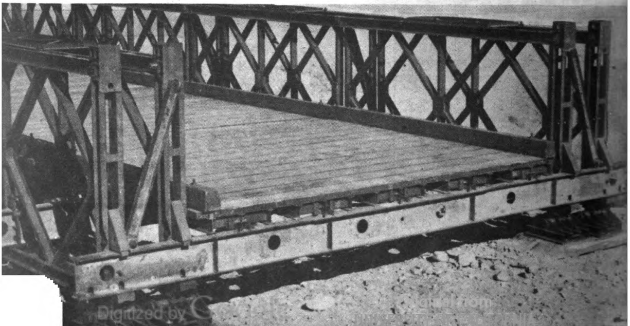
Figure 57.—End of bridge jacked down on bearings.
