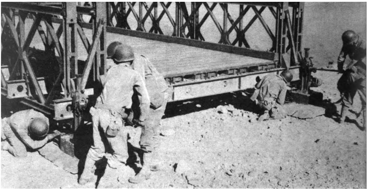
Figure 56.—Jacking down end of bridge on bearings.
