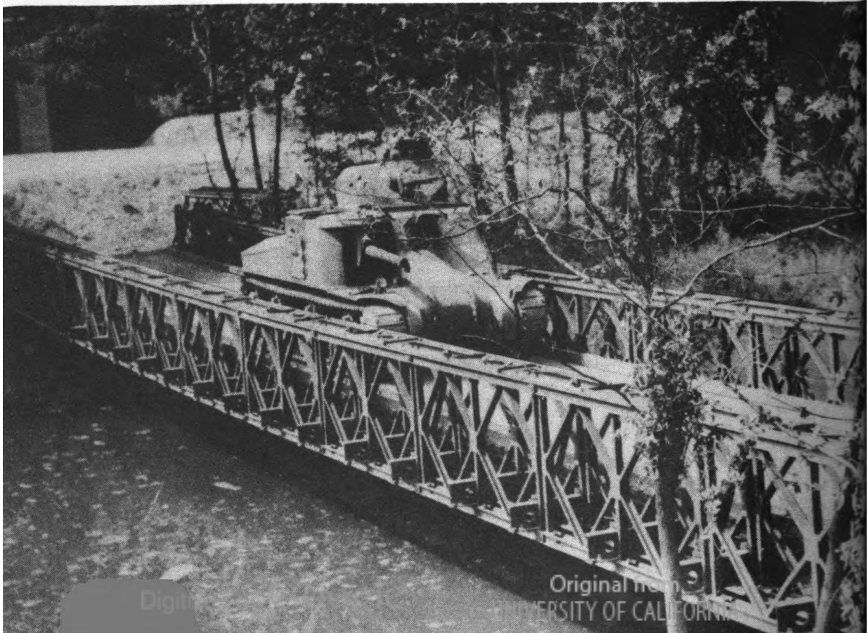
Figure 1.—Medium tank crossing 100-foot double-single bridge.
