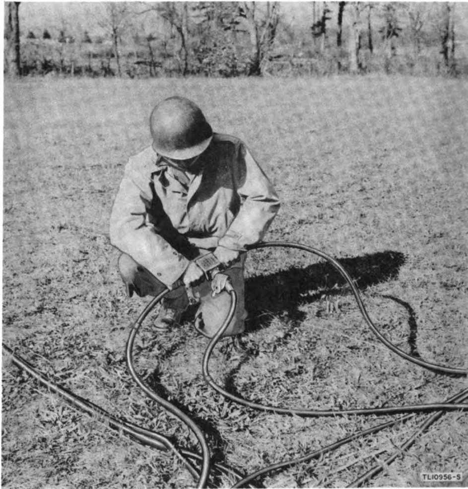
Figure 34. Installation of Junction Box JB-91-A.
