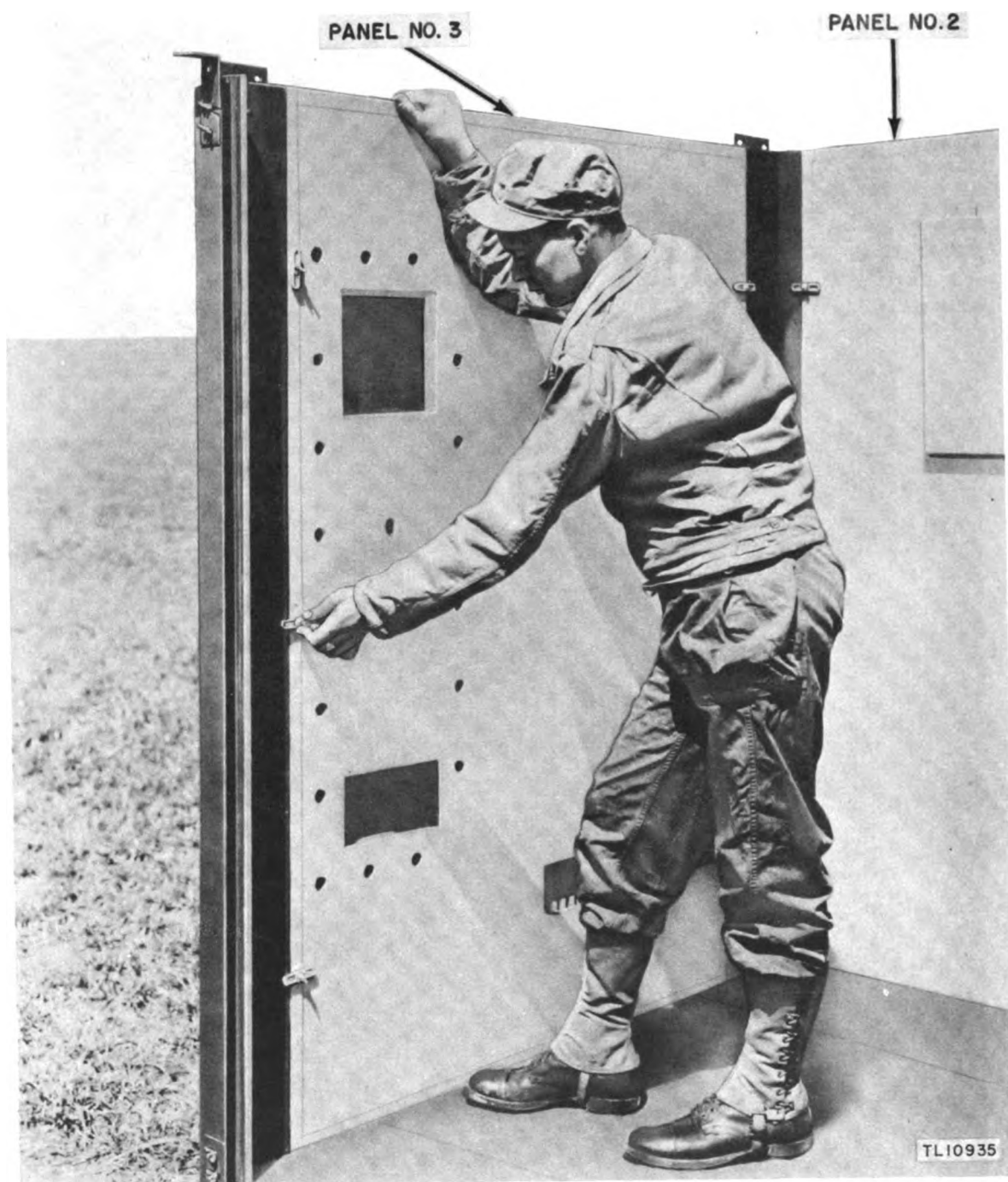
Figure 27. Fastening panel in place.
