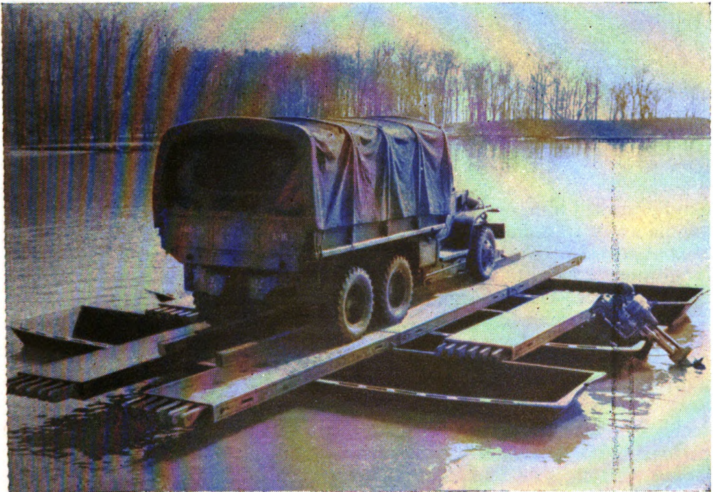
Figure 30. Outboard motor attached to infantry raft using M2 assault-boat bracket.
