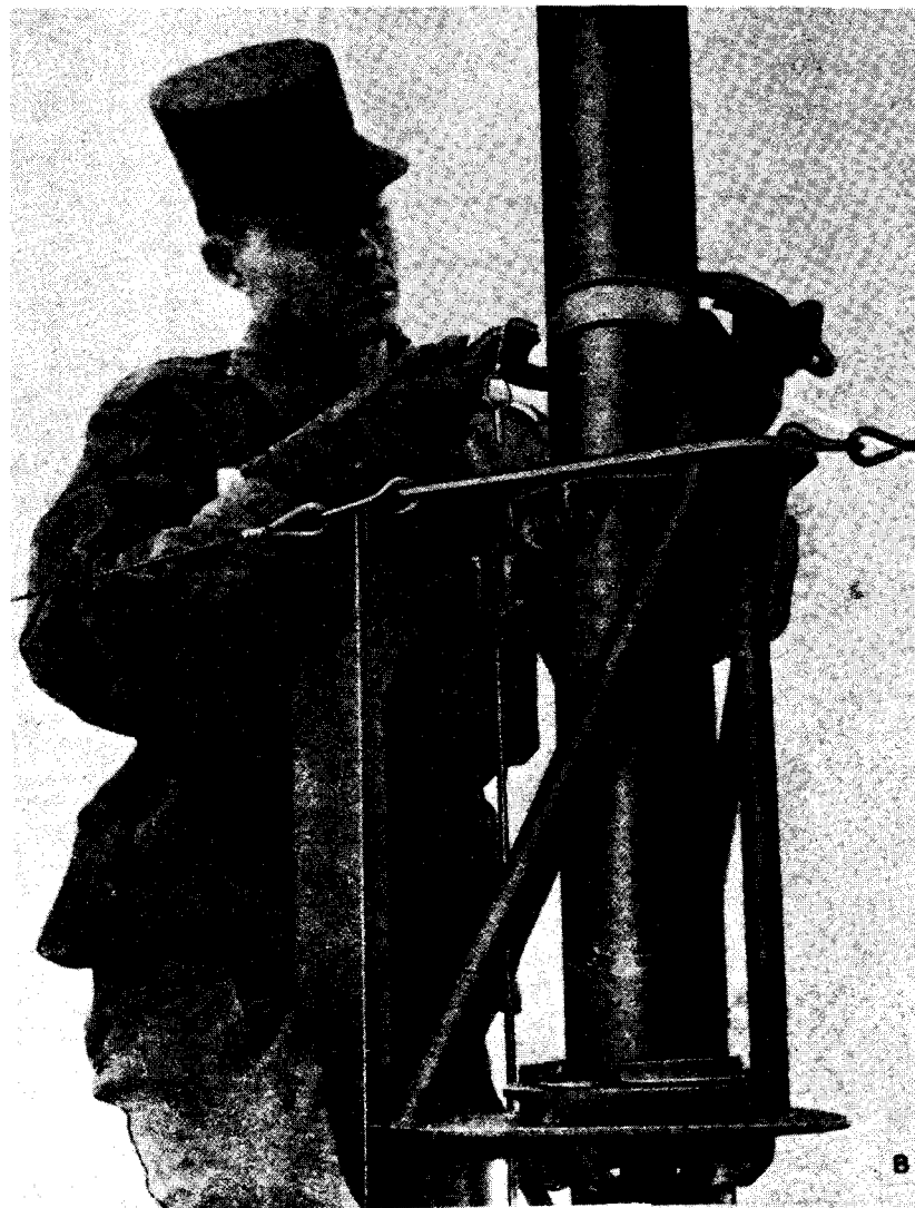
Figure 2-19②. Raising mast (part 2 of 4).
