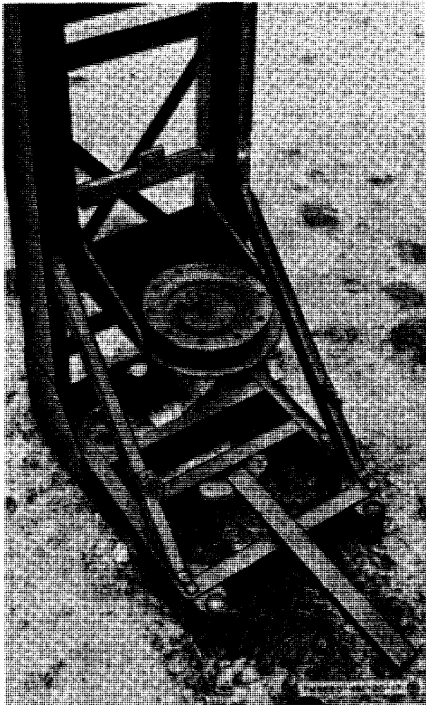
Figure 2-17Ⓣ. Erection of launcher (part 9 of 9)
