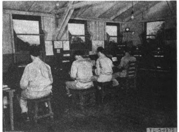
Figure 11-30. Theater signal center operating room with teletypewriter switchboards.
