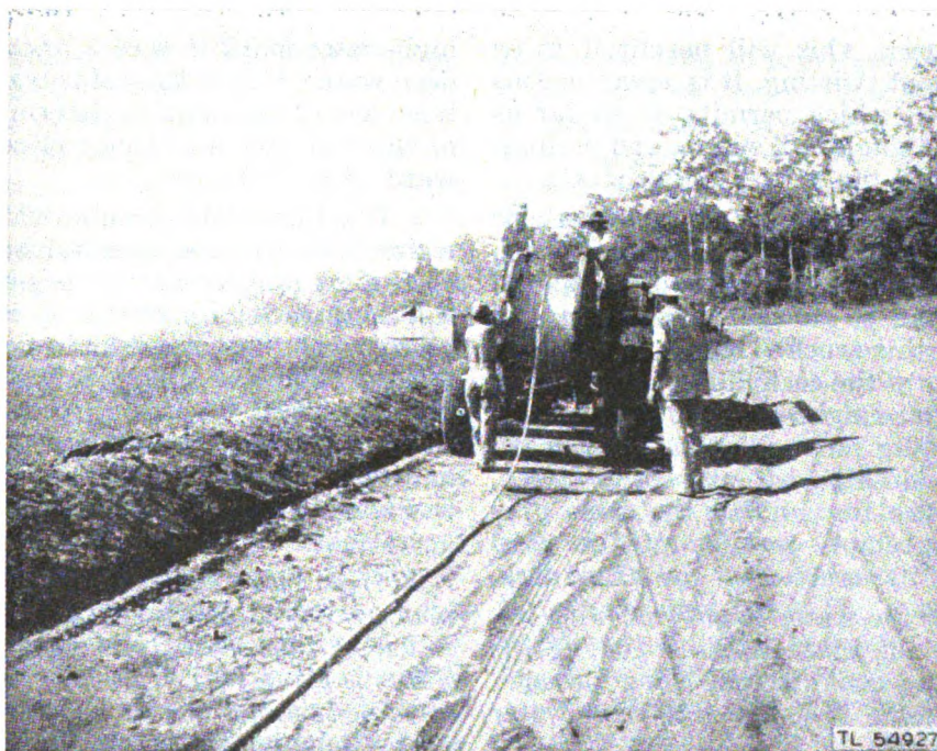
Figure 9-23. Laying lead-covered cable.
