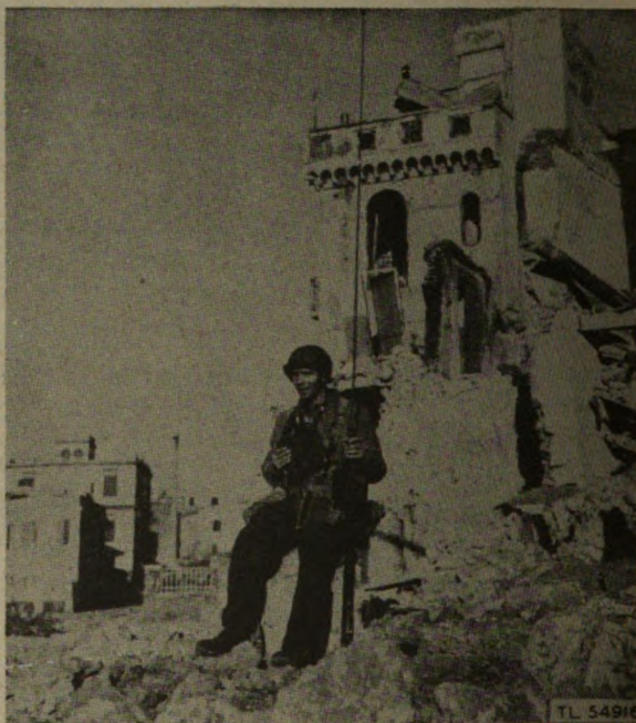
Figure 6-79. Radio Set SCR-511 in operation.
