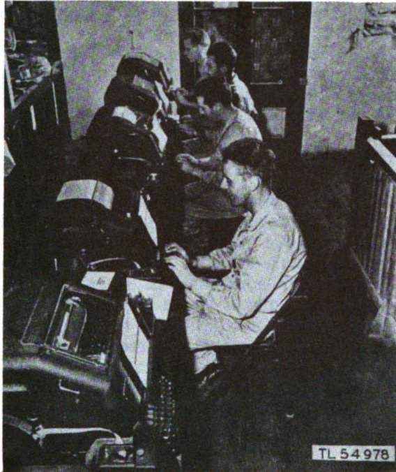
Figure 11-24. Installation of teletypewriter equipment at an operational base.
