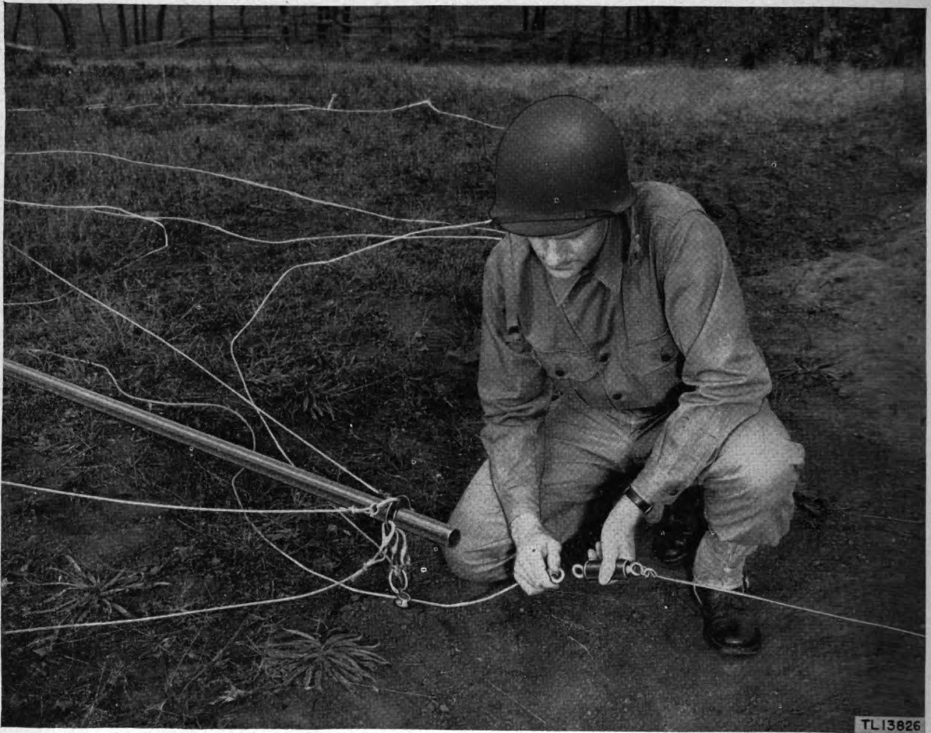
Figure 21. Radio Set AN/MRC-1—receiving antenna wire connection.
