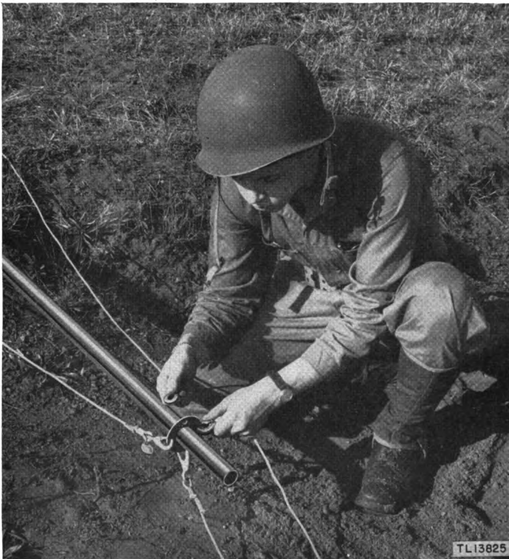
Figure 20. Radio Set AN/MRC-1—receiving antenna guy clips.
