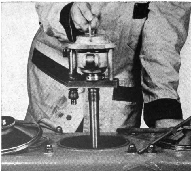
FIG. 17—Lifting Out Injector Assembly
